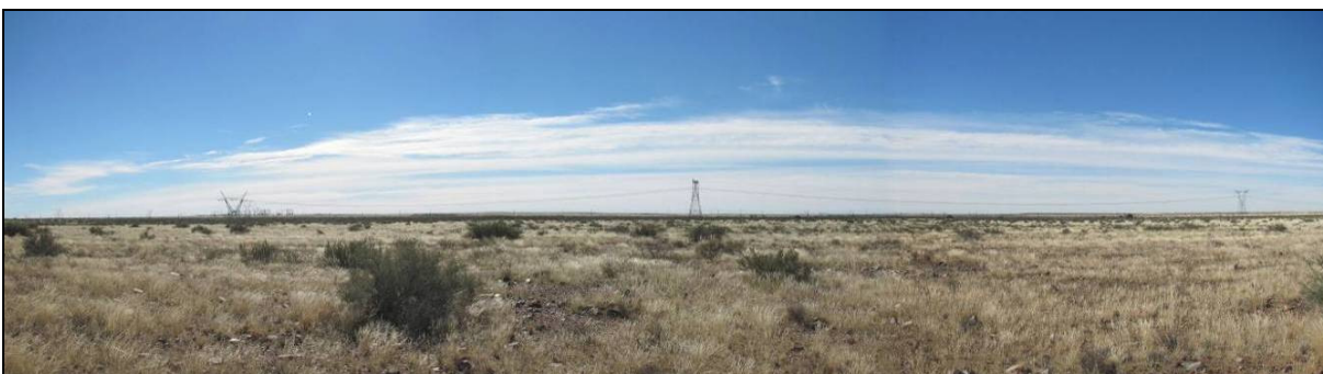
Plate 2: Looking north towards the powerline that crosses the site. Aries sub-station visible on the skyline at left behind a pylon.
