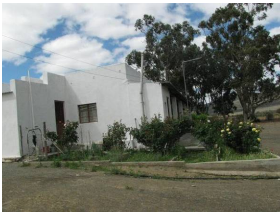
Figure 16 Flat roofed farm house, Haartjieskraal
