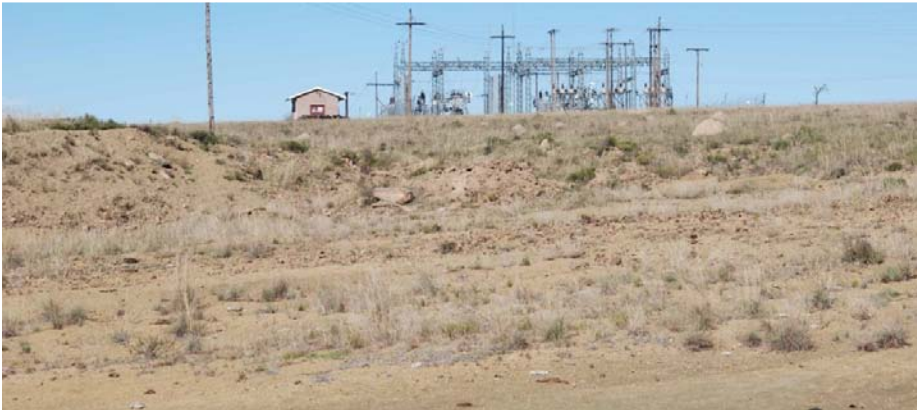
Figure 6: Balfour Formation mudstones exposed in a dam (visible in figure 2) north east of the substation.
