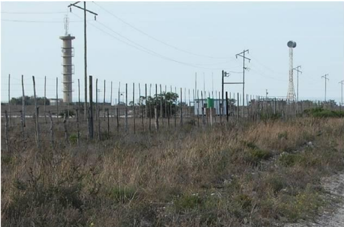
Plate 5-8: Communications towers as seen from site CVP017 at the PPC mine entrance.
