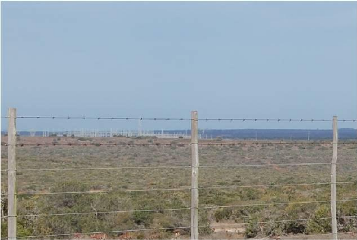
Plate 5-7: A substation as seen from the R335, site CVP016.
