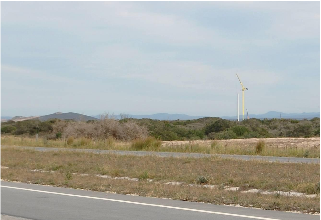
Plate 5-16: Construction of the existing Coega wind turbine (2km away).
