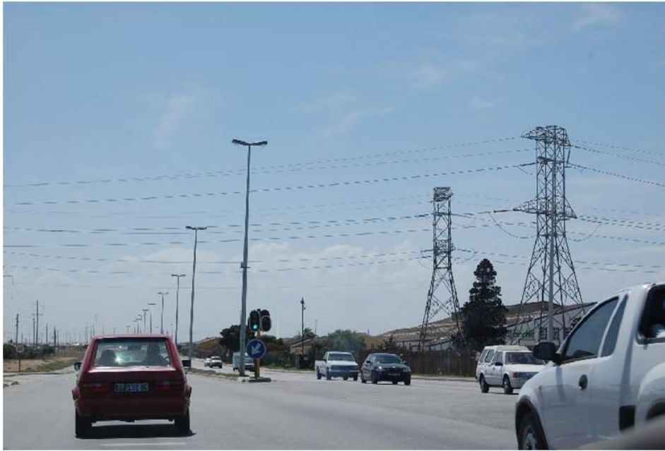
Plate 5-3: Tall power line pylons and street lamps in view at photo site CVP018 near Motherwell.
