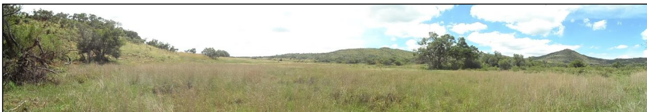
Figure 4-Panaromic view of the dam catchment from the dam wall/embankment
