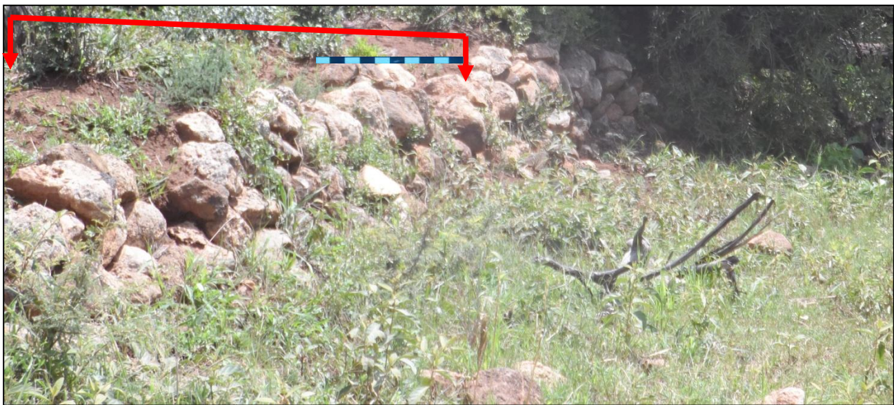
Figure 8- Approximate width of the dam measures between 2m and 2.6m
