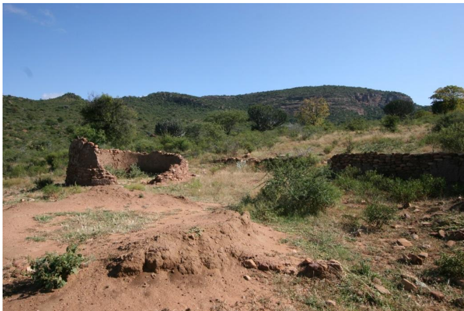
Figure 9: View of existing structures at S.34_05. Note the decaying structure in the left foreground creating typical hut melt. Also note dry packed stone retaining wall to the right of the structures.
