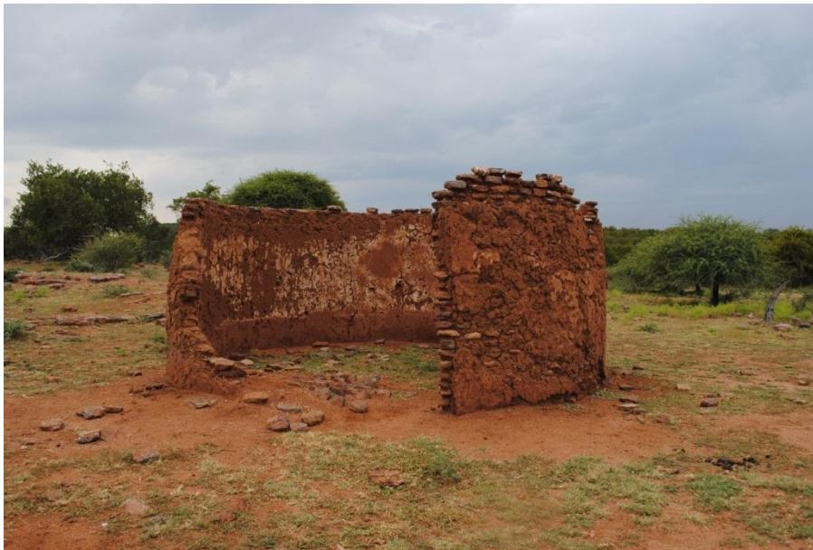
Figure 25: Dilapidated structure and stone foundation in the background at S.34_17
