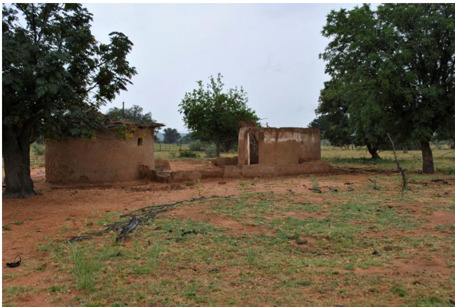
Figure 28: Abandoned structure recorded at site S.34_14.
