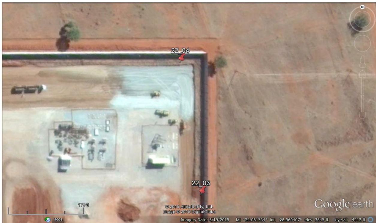
Figure 3: IVN_PGS_22 Test Excavation activities with in the north western corner of the box cut
