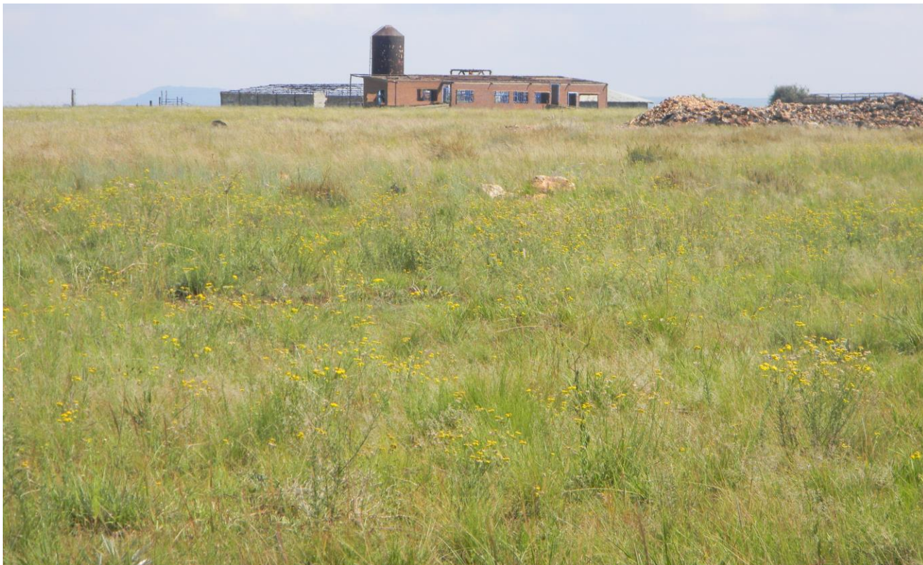
Plate 25: Photo 25: View of abandoned farm buildings and mine diggings on the Farm Wildfontein along Alternative 2A powerline route (Photograph © by Author 2018)
