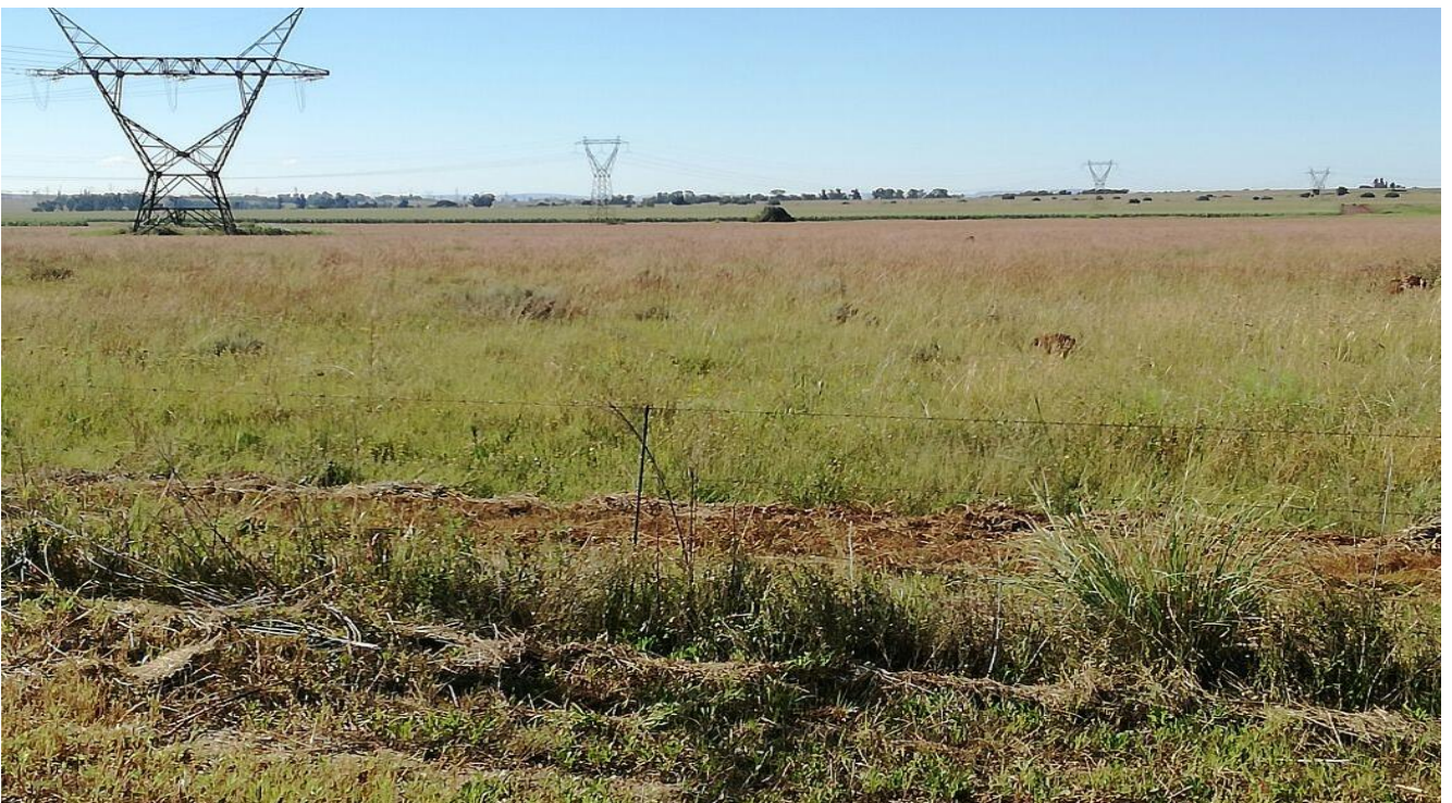
Plate 8: Photo 8: View of existing powerline from Pluto substation to Watershed substation (Photograph © by Author 2018). Note that the proposed Alternative 2 route will run parallel to the existing 400kv line
