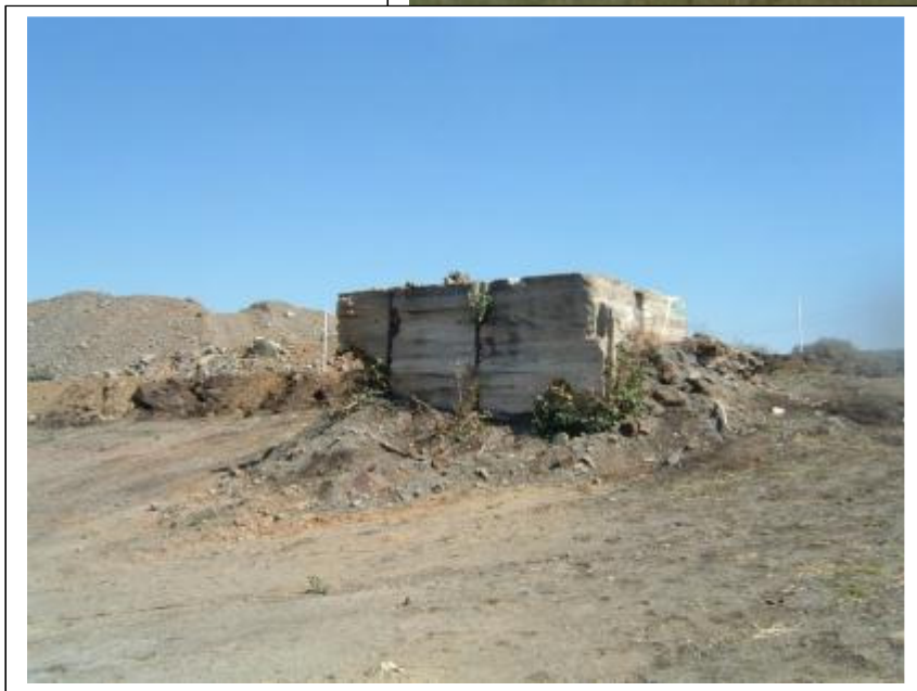
Figures 18, 19 & 20- An incline shaft running into a chrome mine (above). Anchor concrete block on which the mine's head gear rested (centre) and pulleys with cables which hoisted coco pans from the underground mine to the surface where the chrome ore was stock-piled (above).
