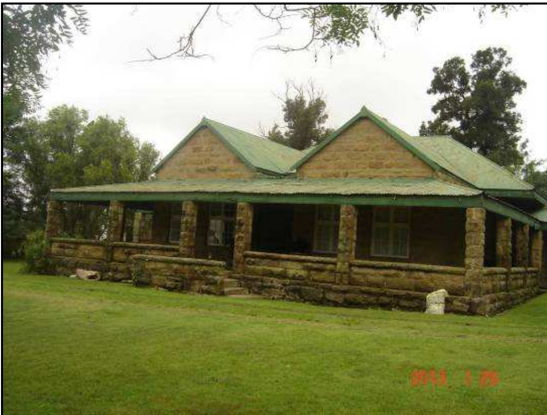
Plate 11: Structure A – Botes Farm House (Portion 13 of farm Zandfontein 74 HS)
