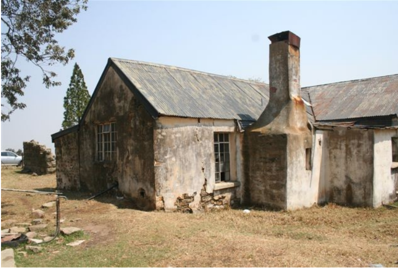
Fig 2: Showing rear portion, with suspected original building and kitchen chimney.
