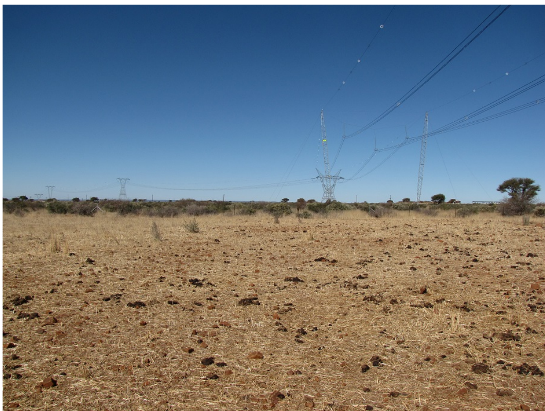
Figure 18: Site 6 facing south
