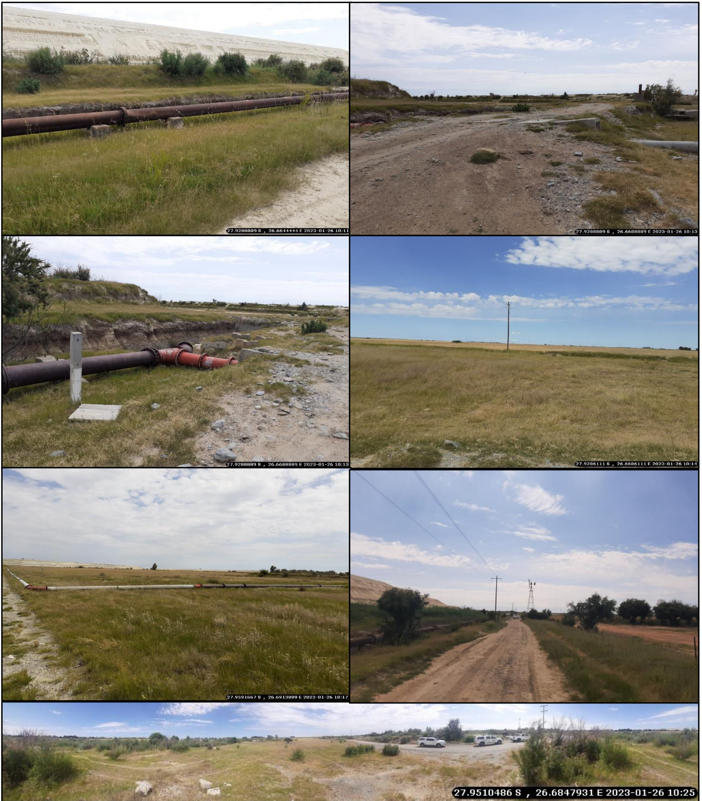
Figure 7: View of the development.
