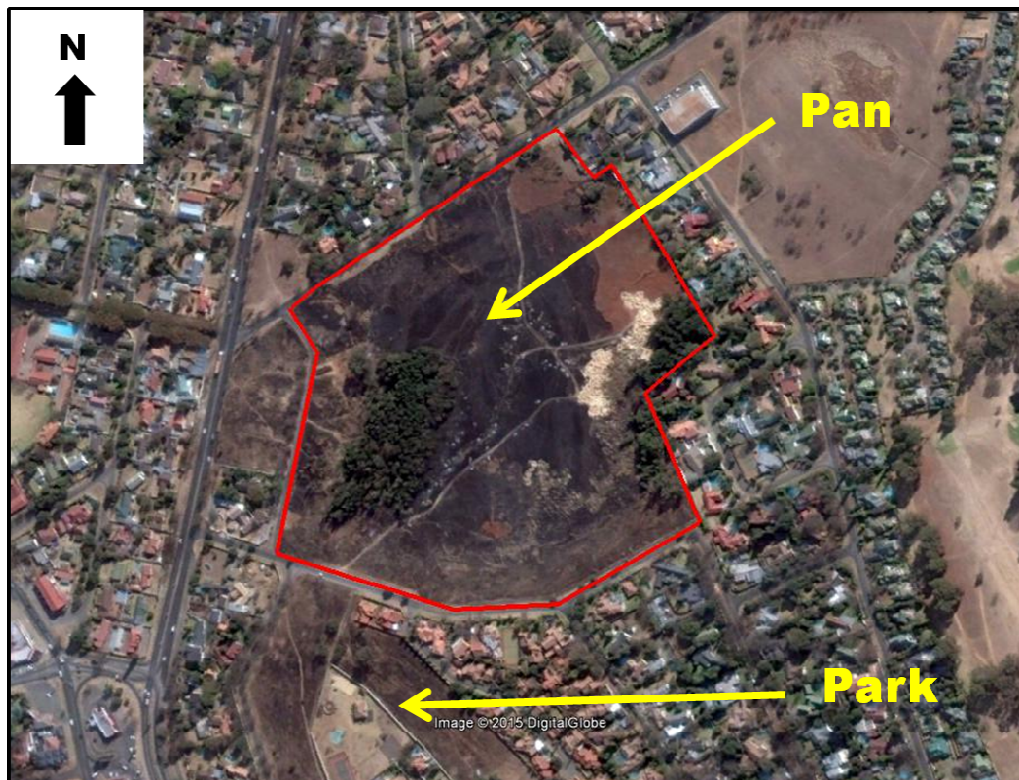
Figure 4: Google earth image of the site of the proposed Morehill Extension 11 Township (red polygon) and its immediate environs.
