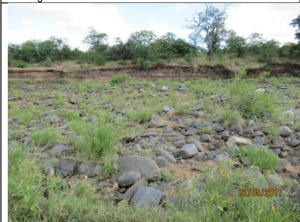
Area at Shangoni Gate where new bridge crossing over the Shingwedzi river will be.
