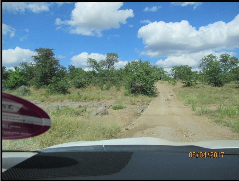
Figure 10: View towards river crossing at the Tshanga Tributary low water bridge crossing.
