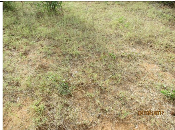
View of shoulder of road at the 10 km mark. The road reserve will be 13.5 m.
