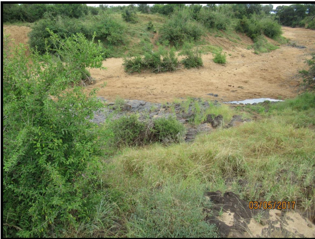
Figure 11: View towards river crossing at the Shingwedzi River, this will be a new bridge crossing.
