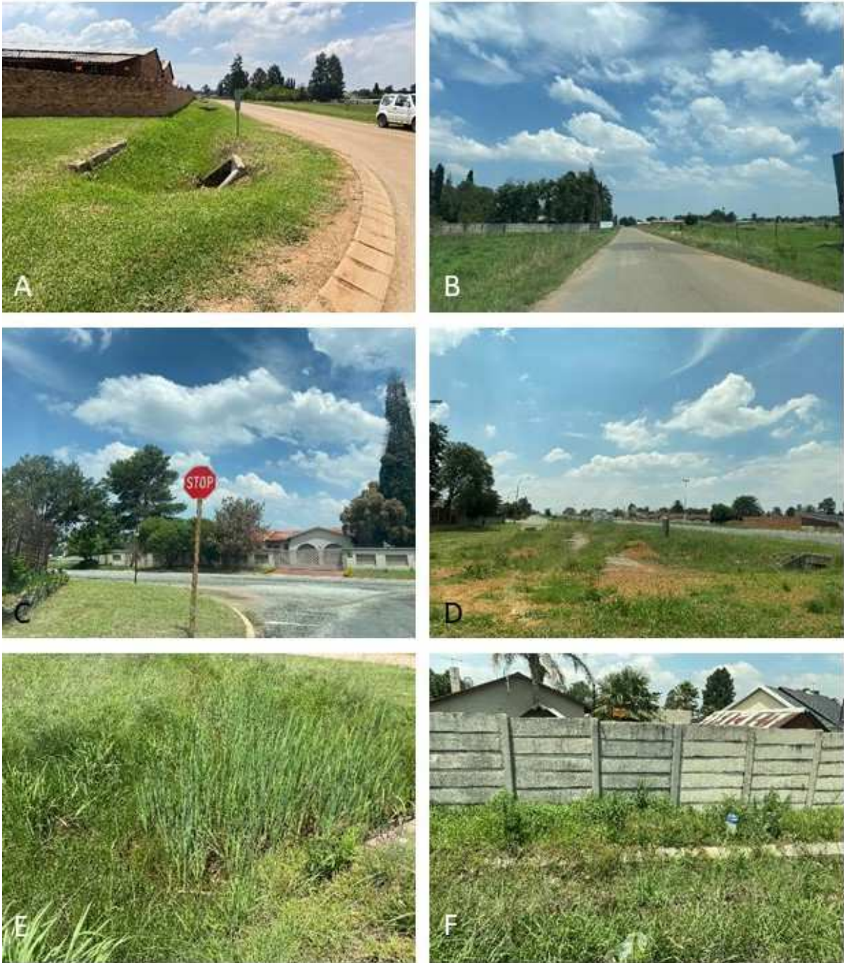
Figure 10: Site visit photographs for the ORTIA SEZ BWS – south and southwestern Bonaero Park in the southwestern extent of the project. See table 3 for road names and observations.
