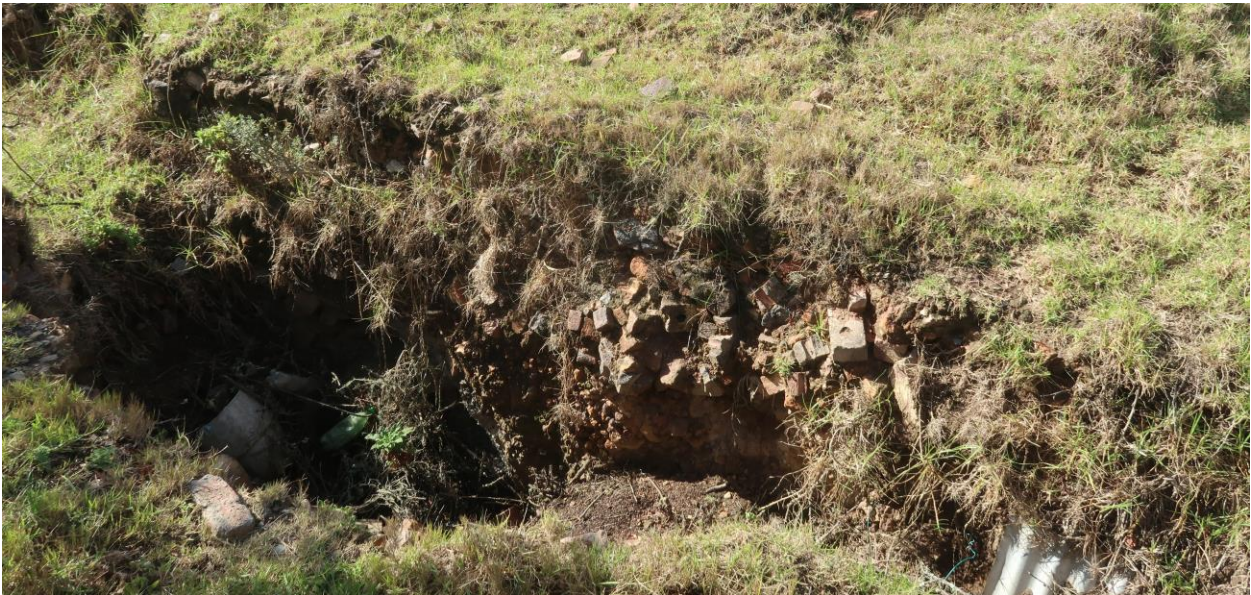
Figure 8: Hole near point 2 (Fig. 4), revealing deep fill of bricks and soil.
