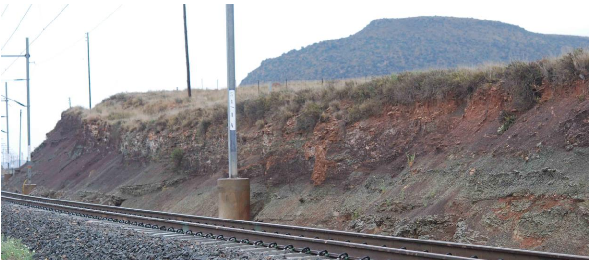
Figure 8: Greenish Balfour Formation mudstone underlying the purplish mudstone in the south east of railcut 2.
