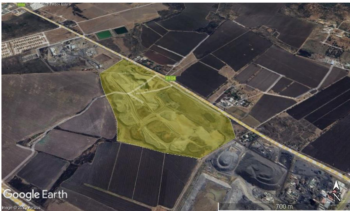
Figure 1: Google Earth site map of the Waterkloof Opencast Mine (yellow polygon) that is under a S24G application.
