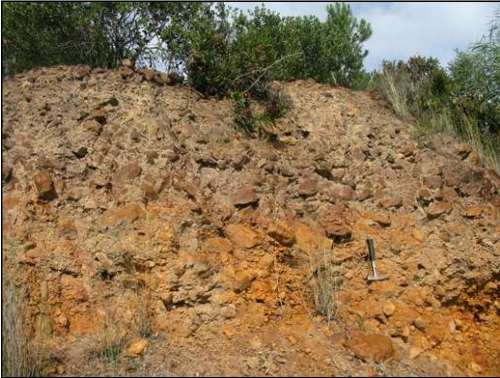
Fig. 17. Thick, blocky ferricretised breccias in road cutting on Diep Rivier's Mond 358 (Loc. 599) (Hammer = 29 cm).
