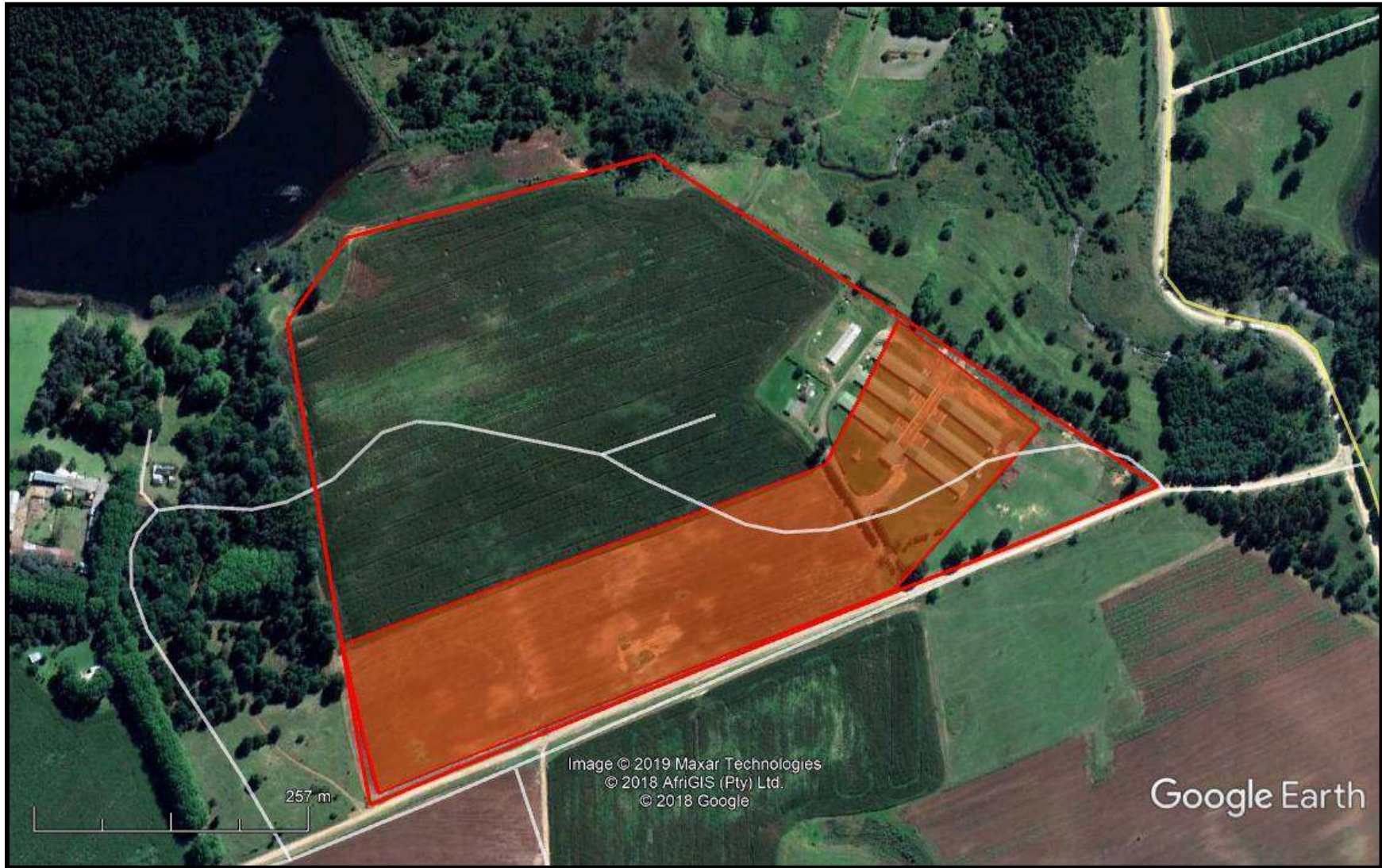
FIG. 2: AERIAL OVERVIEW OF THE PROPOSED DEVELOPMENT
