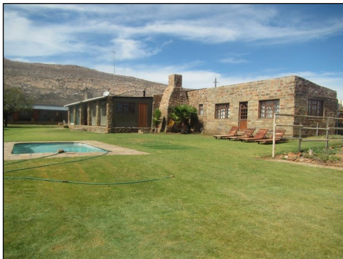
Figure 37: View of the main house. The scale is in 10cm increments
