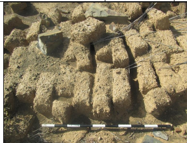
Figure 51: Closer view of the mud and grass bricks used. The scale is in 10cm increments
