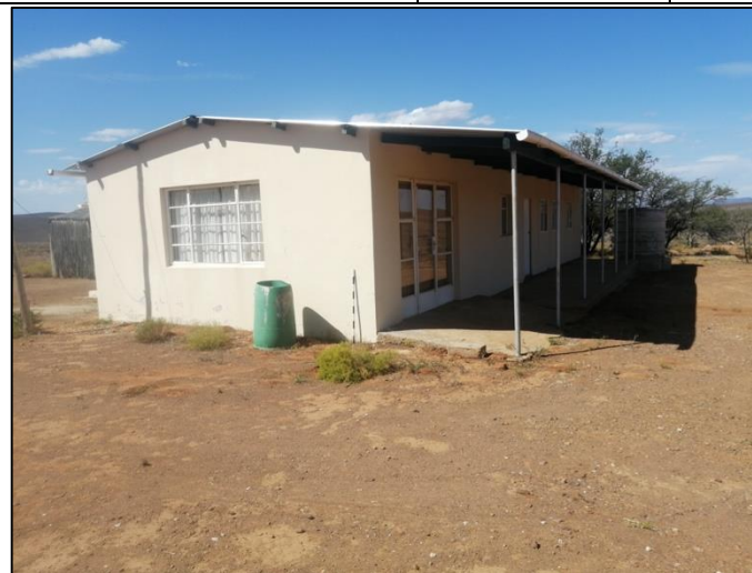
Figure 72: View of the main house. Photo was taken from the south-west. The scale is in 10cm increments.
