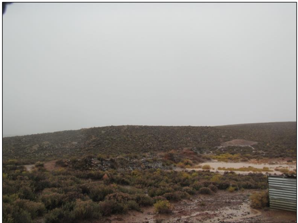
Figure 87: View of the dam wall at site PK 19.
