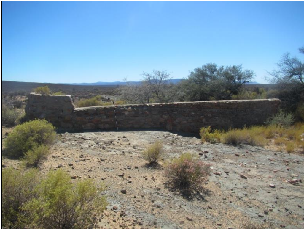
Figure 32: View of the stone wall at site PK 04.
