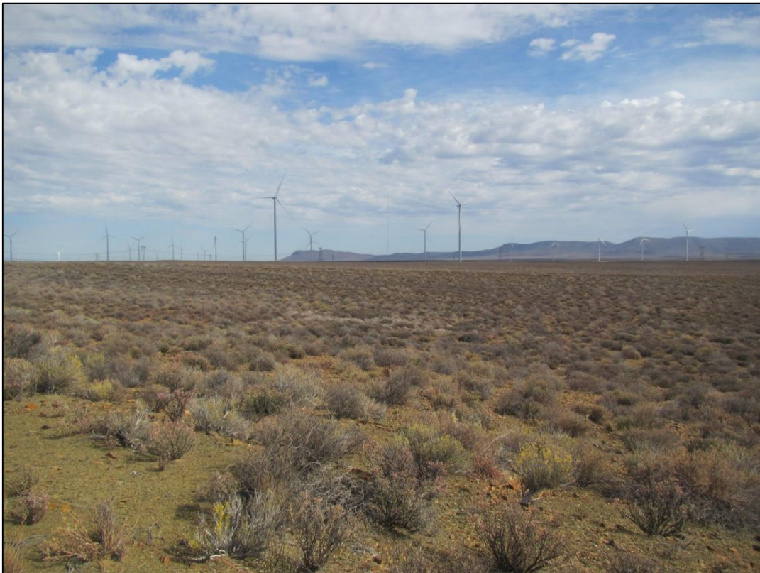
Figure 16: View of existing turbines.
