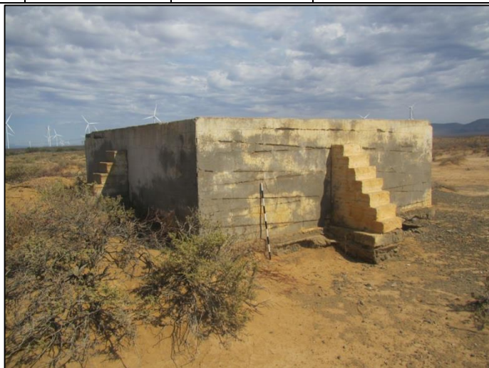
Figure 96: View of the reservoir. The scale is in 10cm increments.
