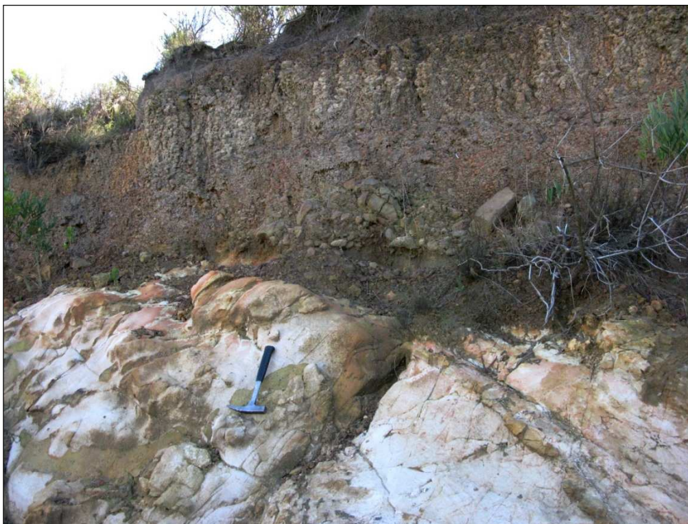
Fig. 22. Downwasted gravels, nodular ferricrete and silty soils overlying weathered Cederberg Formation mudrocks, borrow pit along R332 (Loc. 085).
