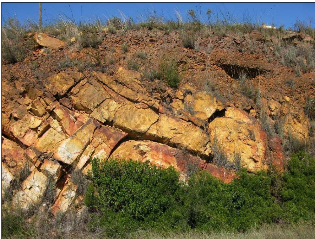
Fig. 18. Rubbly ferricrete gravels overlying gently-dipping, weathered Goudini Formation bedrocks, R330 road cutting NE of Rondebos (Loc. 052).
