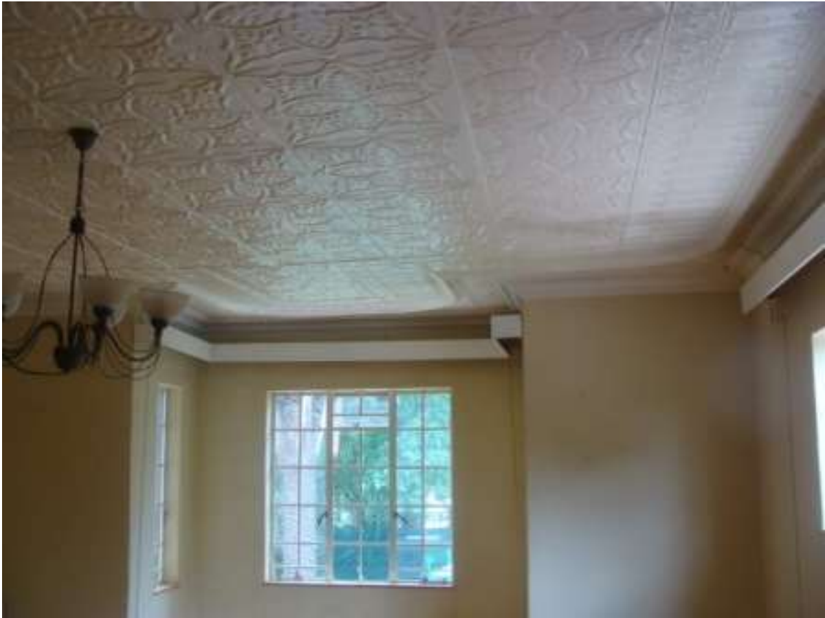
Figure 15: Another room with pressed ceilings. Although these features could be older than 60 years of age, modern renditions are known to exist.
