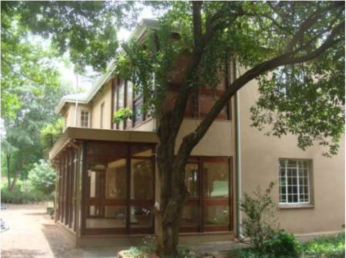
Figure 13: A view of a section of the front of the house. The section with the wooden framing is a modern addition.
