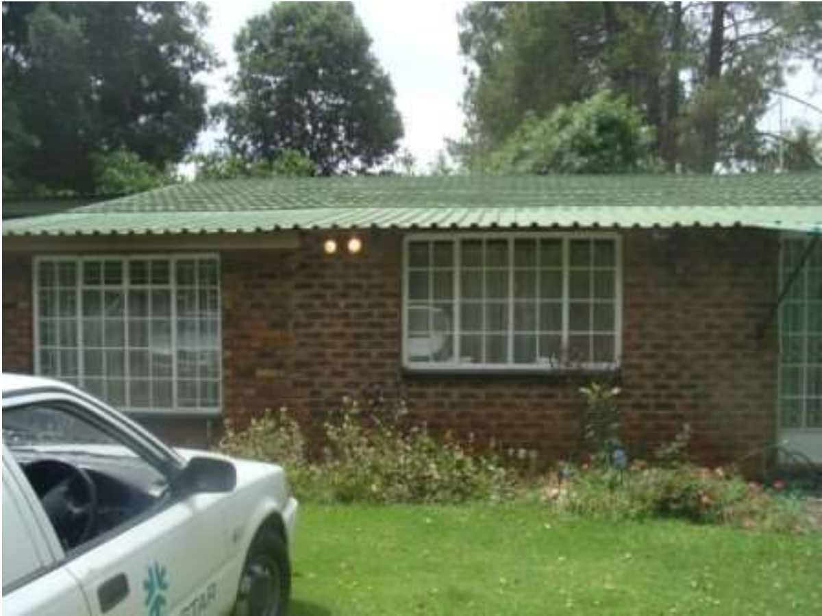
Figure 9: Modern brick structure on the property.
