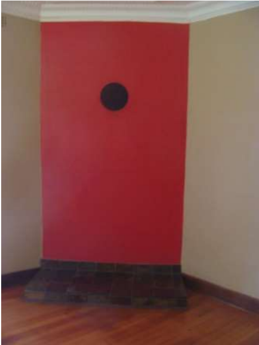
Figure 17: Location of what could have been the original hearth. This has now been closed-up.
