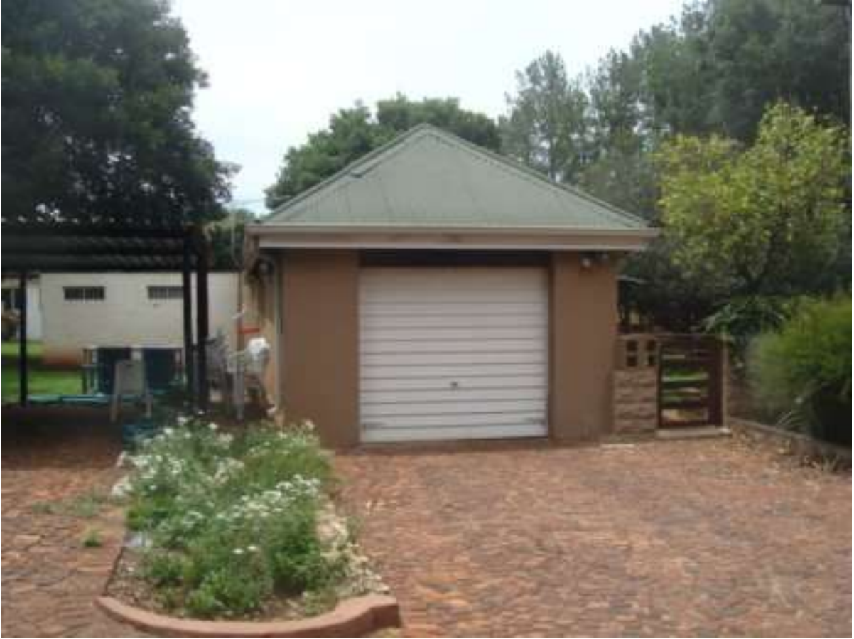
Figure 10: Another outbuilding (garage).
