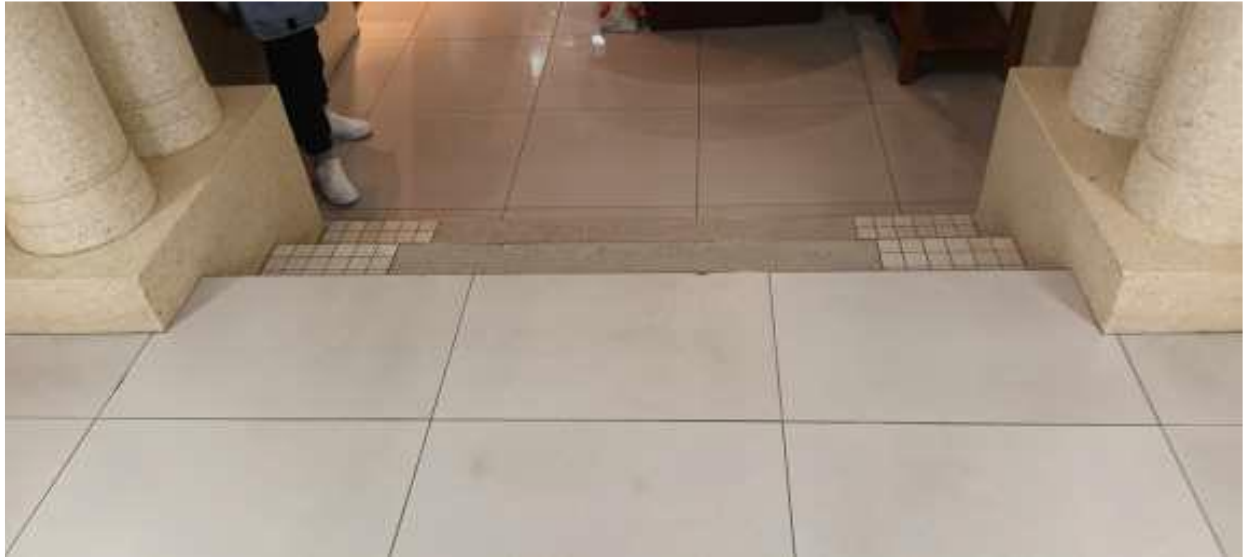
Fig 5 : Main Entrance Lobby : Steps dividing the two lobbies
