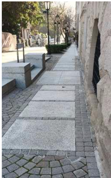
Fig 2 : Existing ramp-up area at the Main Entrance
