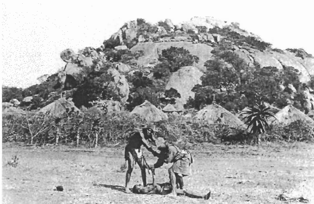
Fig. 20. Photograph taken on the site by H.F. Gros during the 1880s. Although he does not explain the action presented in the foreground, the background gives a clear picture of the last phase of occupation on the site.
