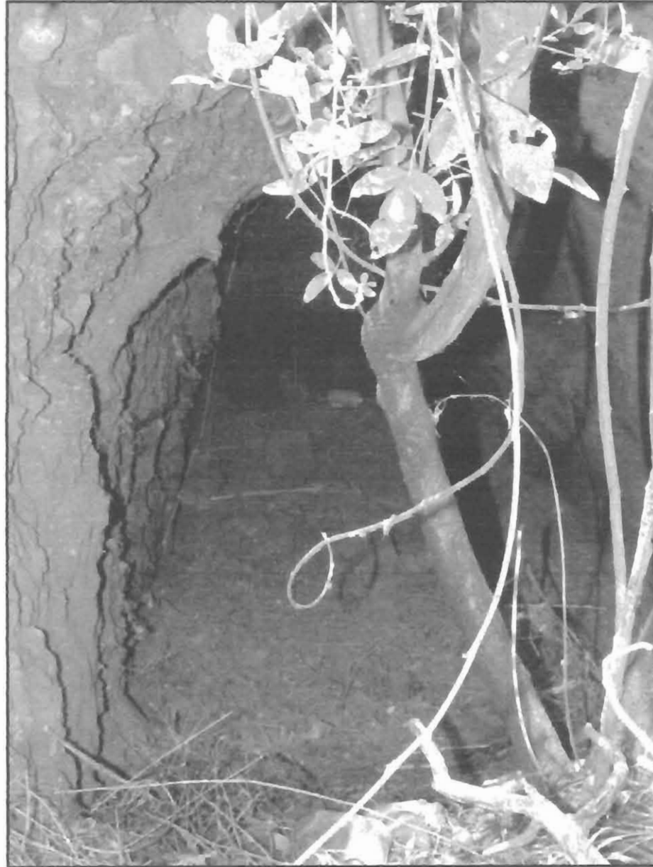
Figure 14 - Entrance to Shaft GR024
