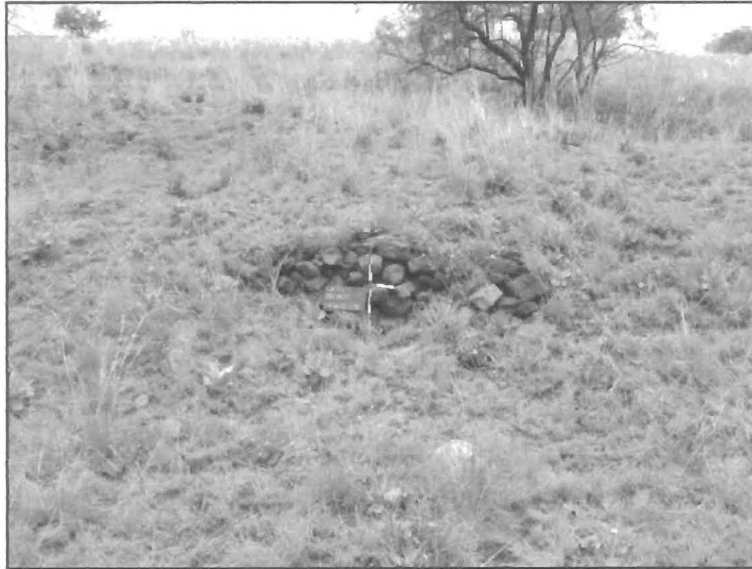
Figure 9 - Low retaining stonewall
