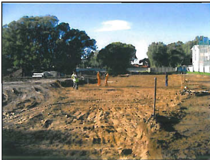
Photograph 5: The box-cut excavations along the route of the Granger Bay Boulevard.
