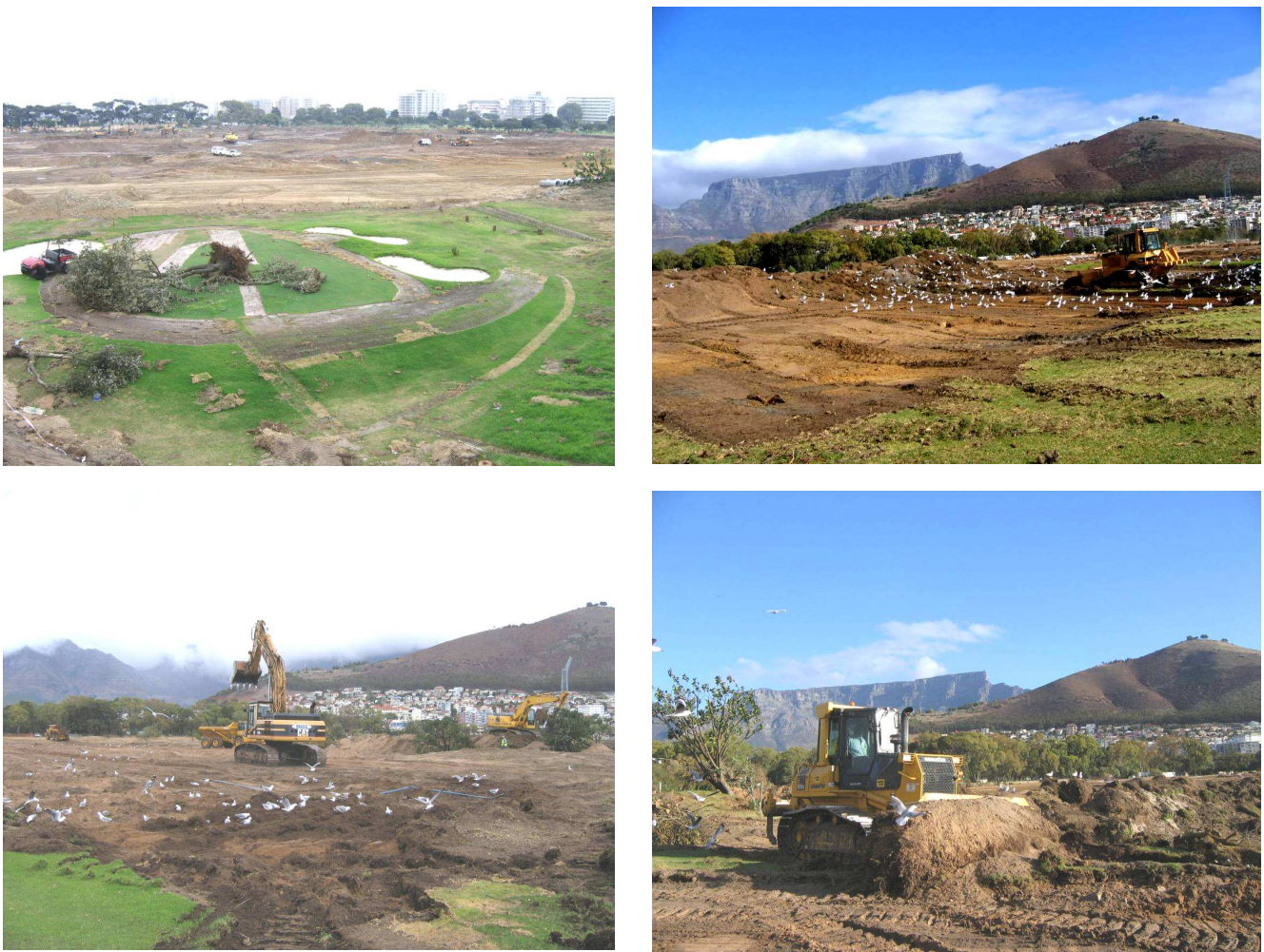
Figure 4 : removal of trees, turf and topsoil from the site
