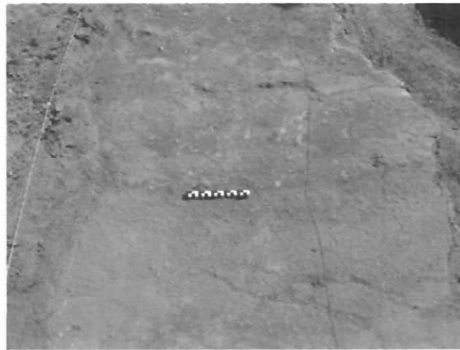
Figure 14. Photograph of the western raised curb.
