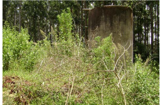
Fig 27: remaining water tower
