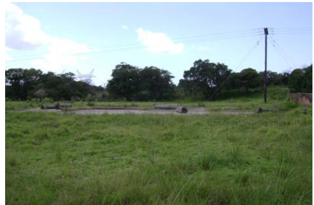
Fig 14: concrete platform and ramp (right)
