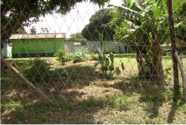
Fig 54: view of ablution block
