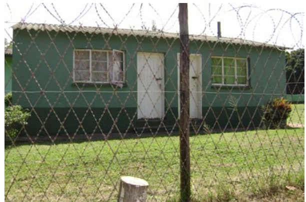
Fig 53: view of unit
