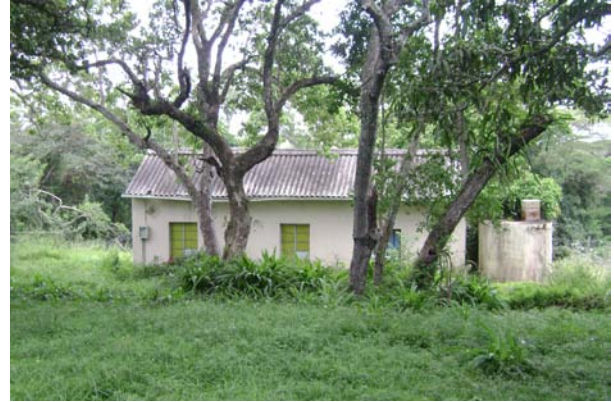
Fig 46: derelict building no 5
