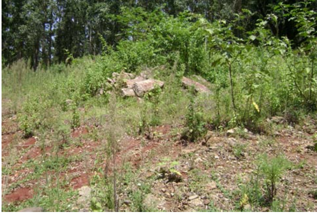
Fig 26: bulldozed foundations with rubble on top
