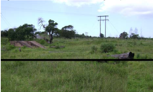
Fig 15: looking towards elevated road level
