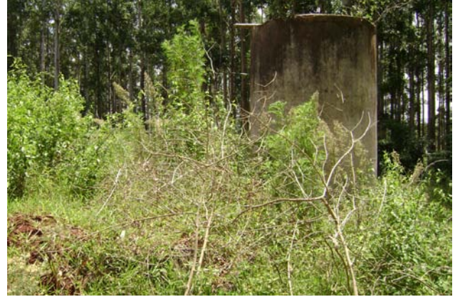
Fig 27: remaining water tower
