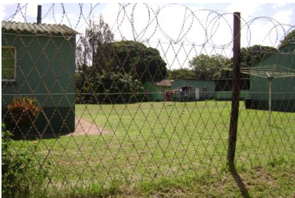
Fig 52: view of group from road
