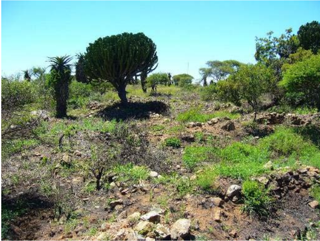
Fig 17. Visual documentation of walling.
