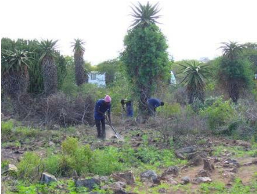
Fig 15. Clearing of walls, manually.
