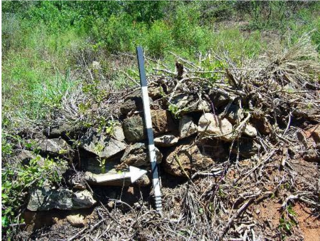
Fig 19. Visual documentation of walling.
