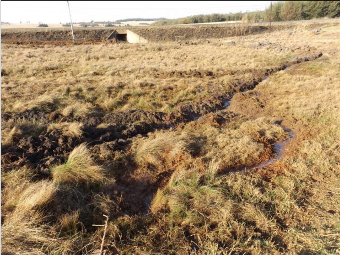
Figure 6: Downstream of the dam wall and upstream of the R33 roadway. This is highly weathered dolerite which has become mud.
