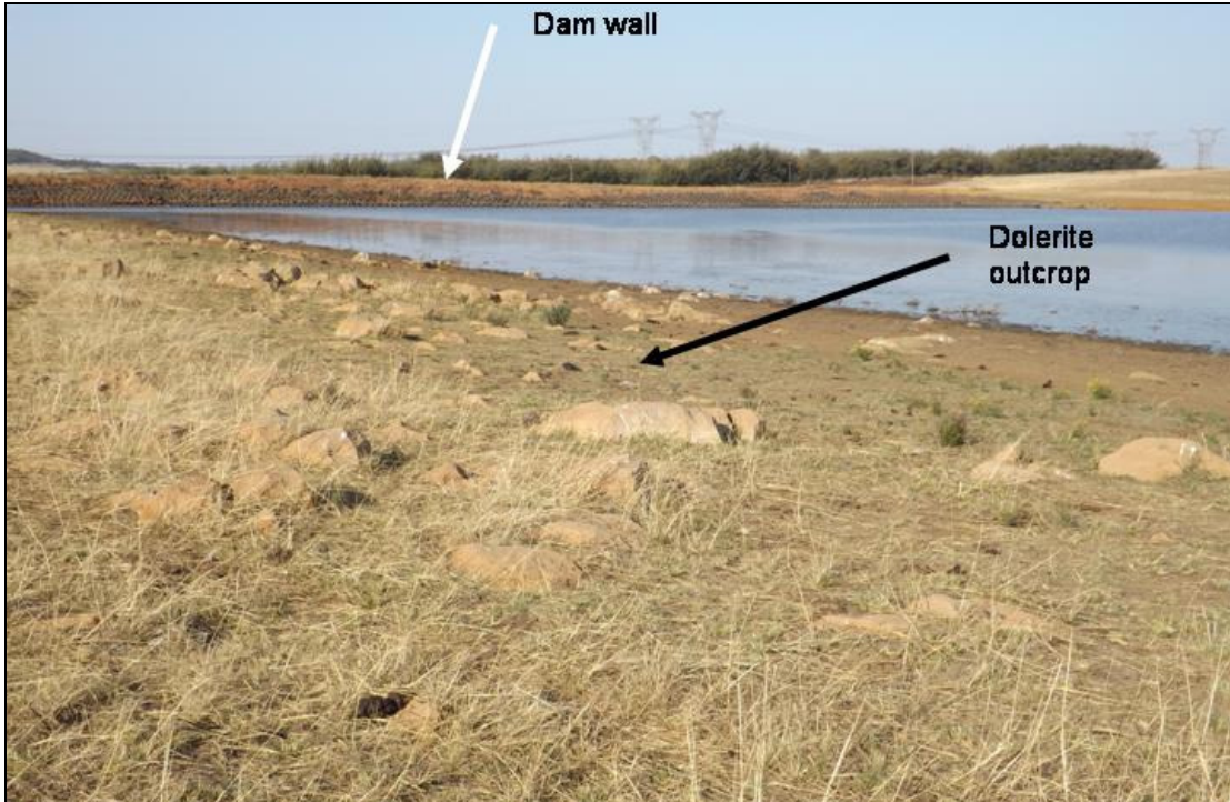
Figure 4: Dolerite outcrop on the left (north) bank of Persberg Dam.
