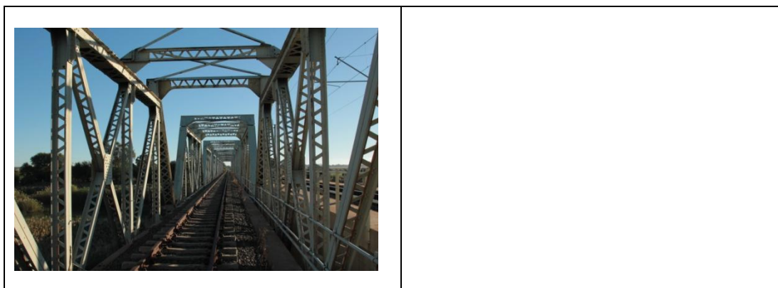
Fig. 8. Infrastructural elements in the environment (bridges and mining features).
