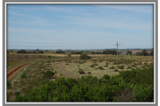
FIGURE 8 LOCATION OF TOWERS 5 AND 6.
