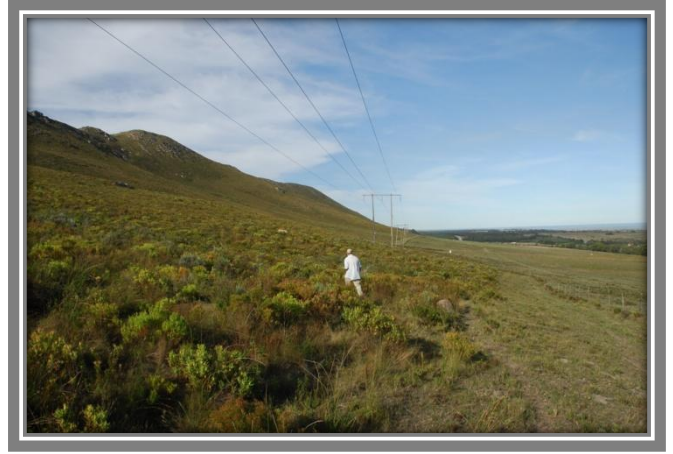
FIGURE 11 VIEW EASTWARDS OF TOWERS 29-32.
