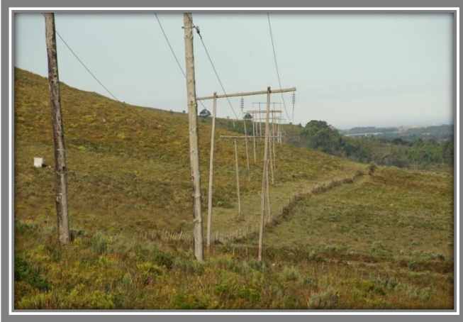
FIGURE 10 VIEW EASTWARDS OF TOWERS 32-35.
