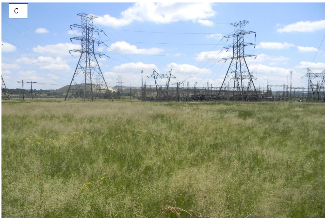
Plate 3: Photo C. showing the Westgate substation site earmarked for expansion..
