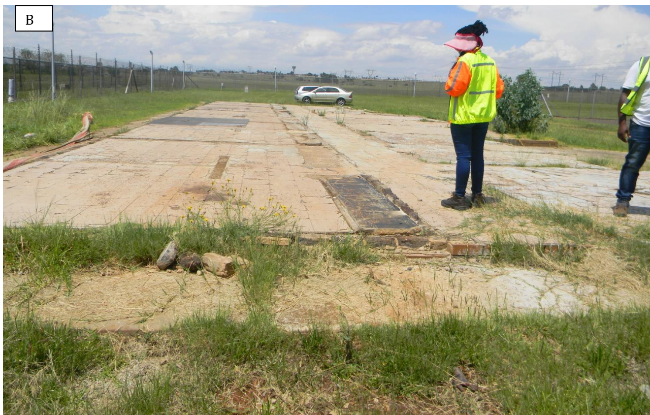
Plate 2: Photo B . showing Eskom and Kimopax officials inspecting the derelict house.
