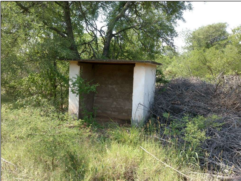
Figure 27: Larger explosives building at site TA02.
