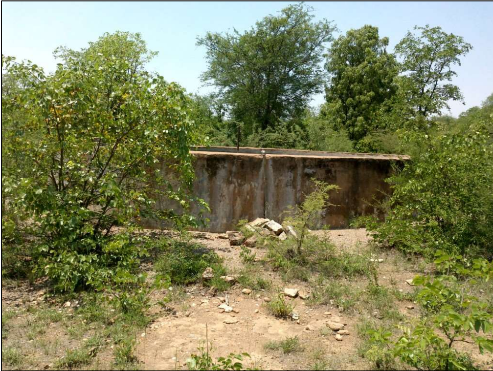
Figure 30: Site TF02 – water reservoir.
