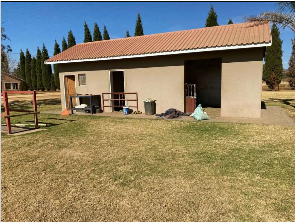
Figure 28: Building at Site K17.
