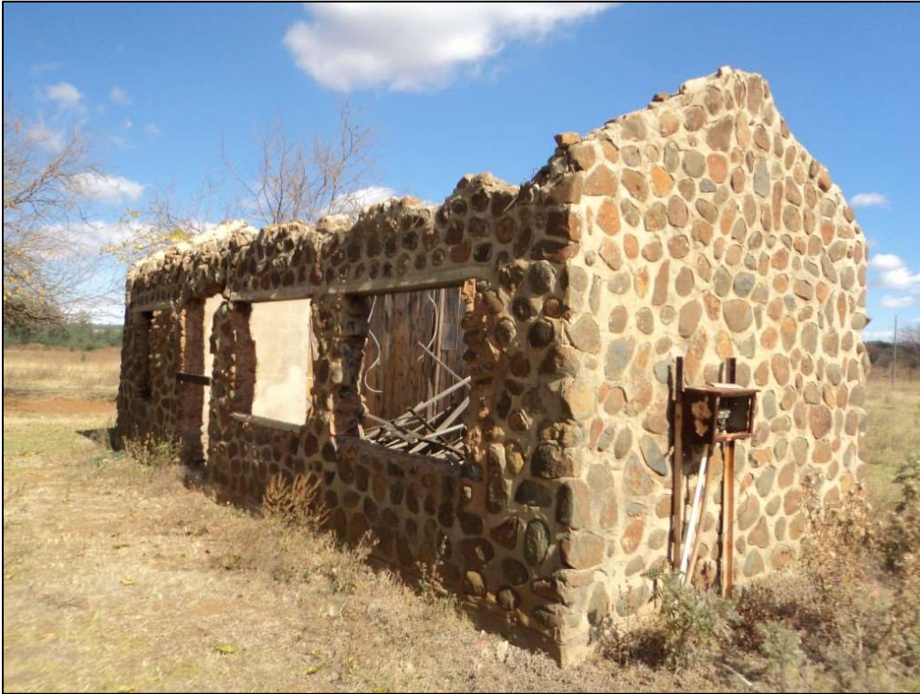
Figure 31: Building ruin at Site K05.
