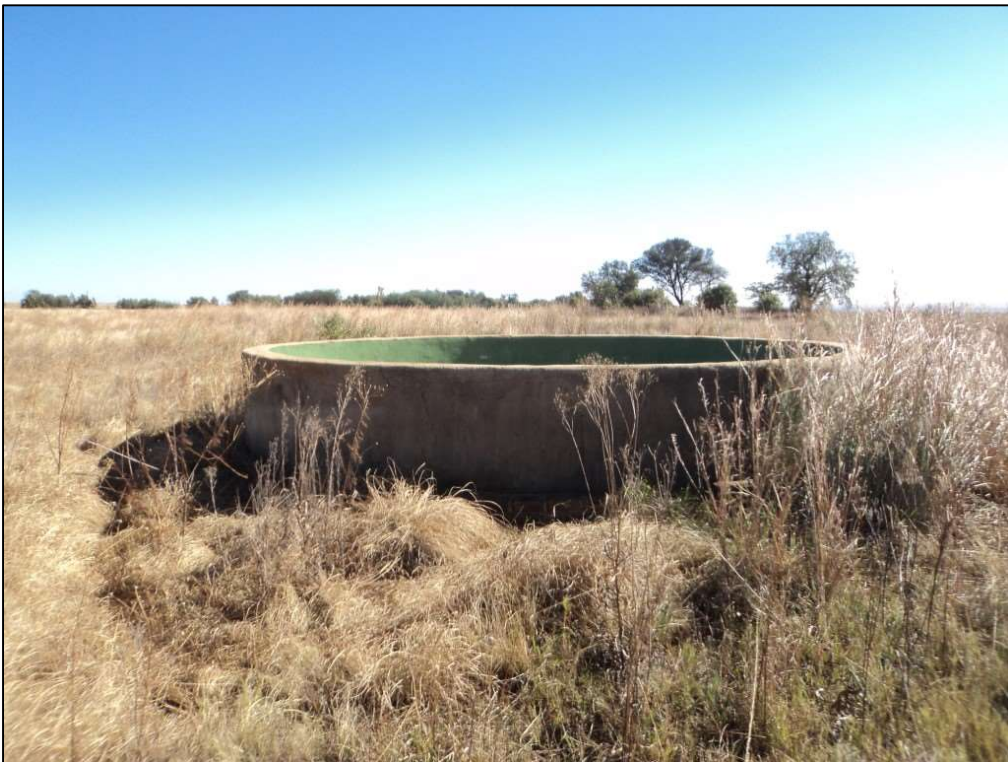
Figure 38: Water reservoir at Site K11.
