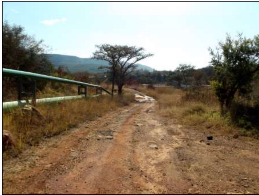
Fig. 22. Site SO 11. Photo taken in a northern direction.
