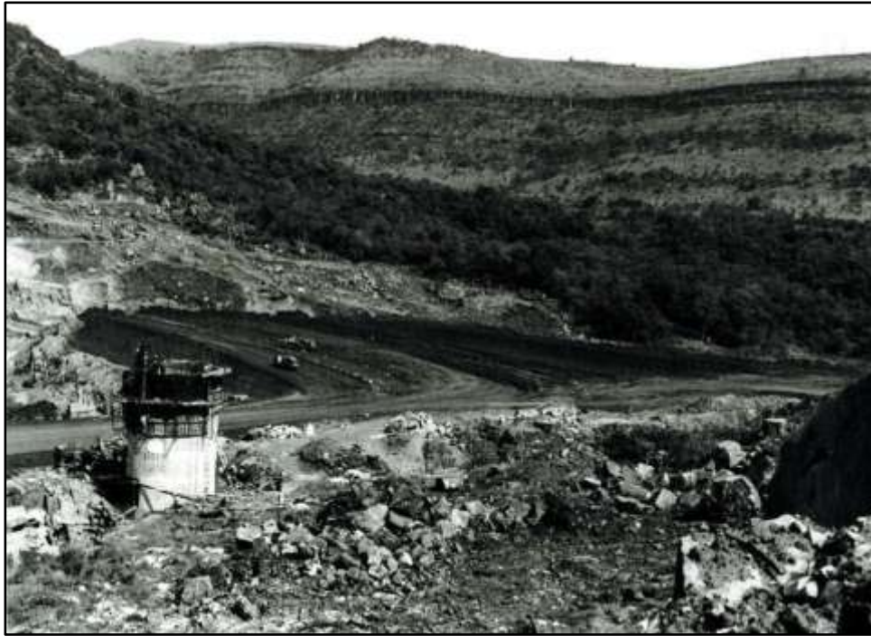
Fig. 4.3. Ngodwana Dam wall construction in 1983 (photo source, Hocking, 1987:263).
