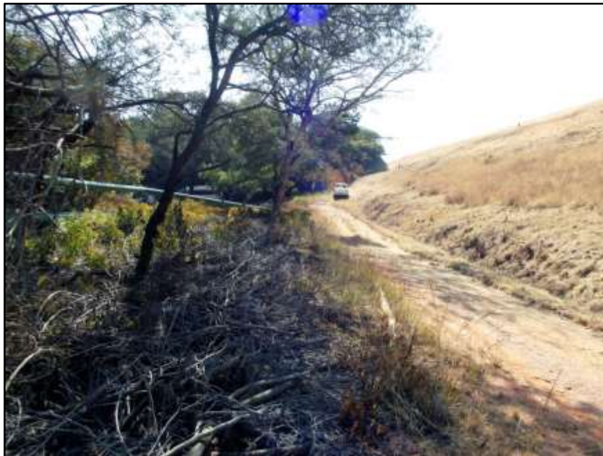
Fig. 14. Site SO 7. Photo taken north. The access road proposed to widen and stabilizing berm to be constructed. To the right is the current dam wall or embankment.
