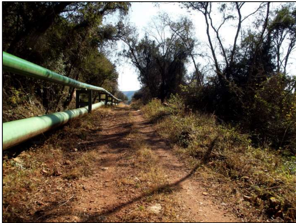
Fig. 18. Site SO 9. Photo taken in a north-western direction. Access road to be widened.
