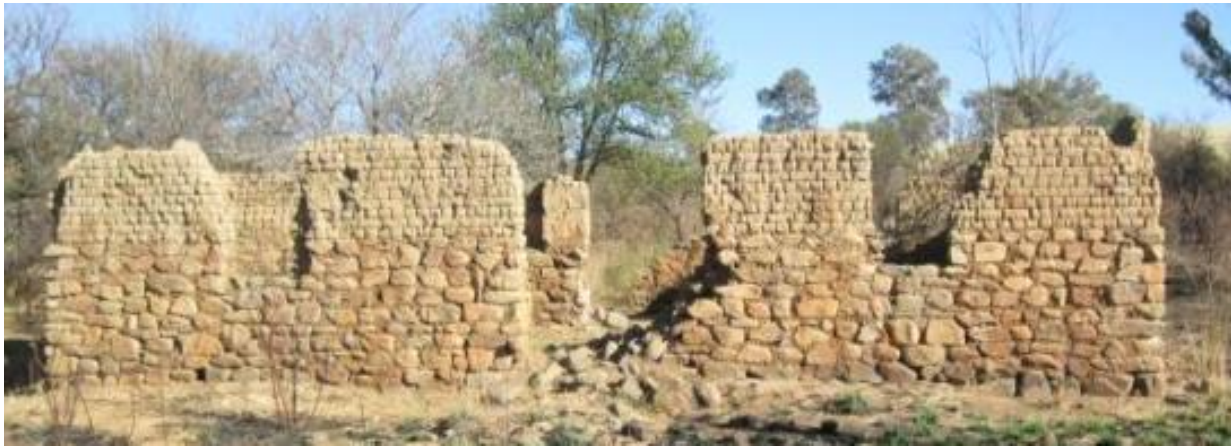
Fig. 06. The remains of one of the Schutte family's dwellings from the 1850s on the farm Deelkraal to the southwest of Johannesburg, which is typical of early pioneer architecture.)
