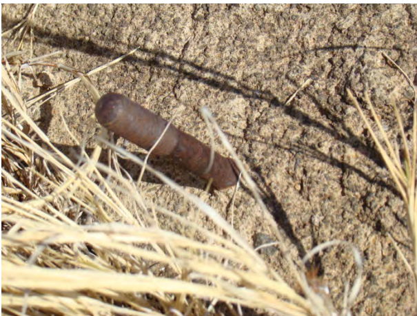
Figure 40: Threaded bolt embedded in concrete foundation
