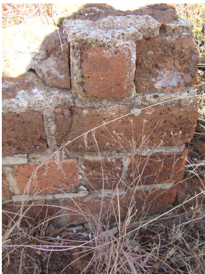
Figure 44: Bricklaying method clearly visible
