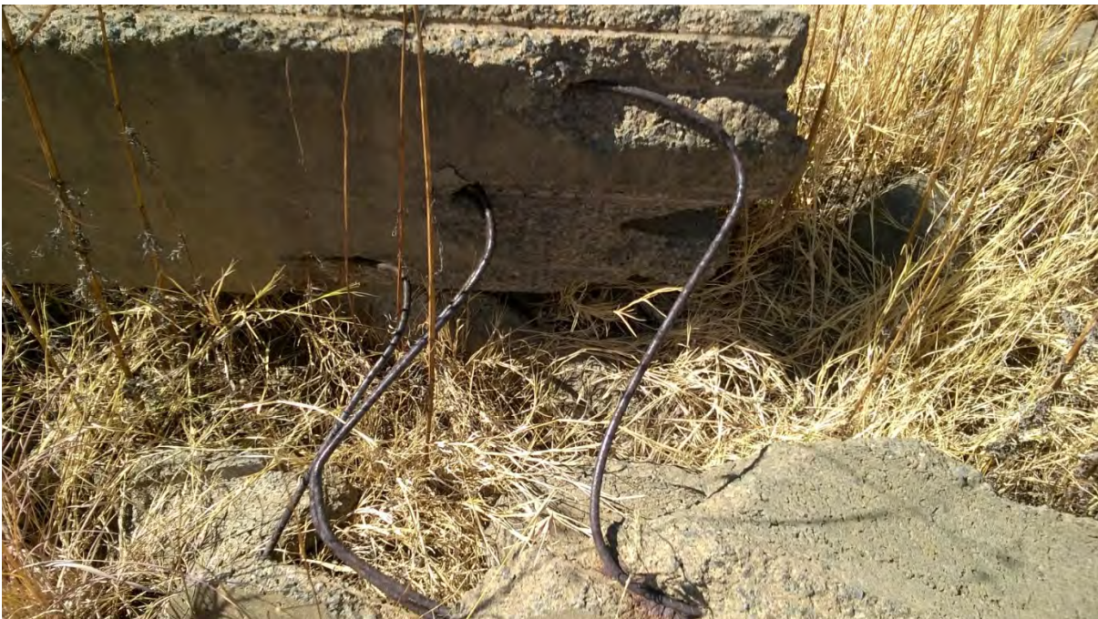
Figure 63: Reinforced concrete remains
