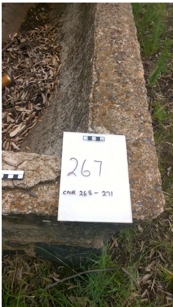
Figure 47: Close-up view of the missing moulding with the thin layer of cement clearly visible on the inside.
