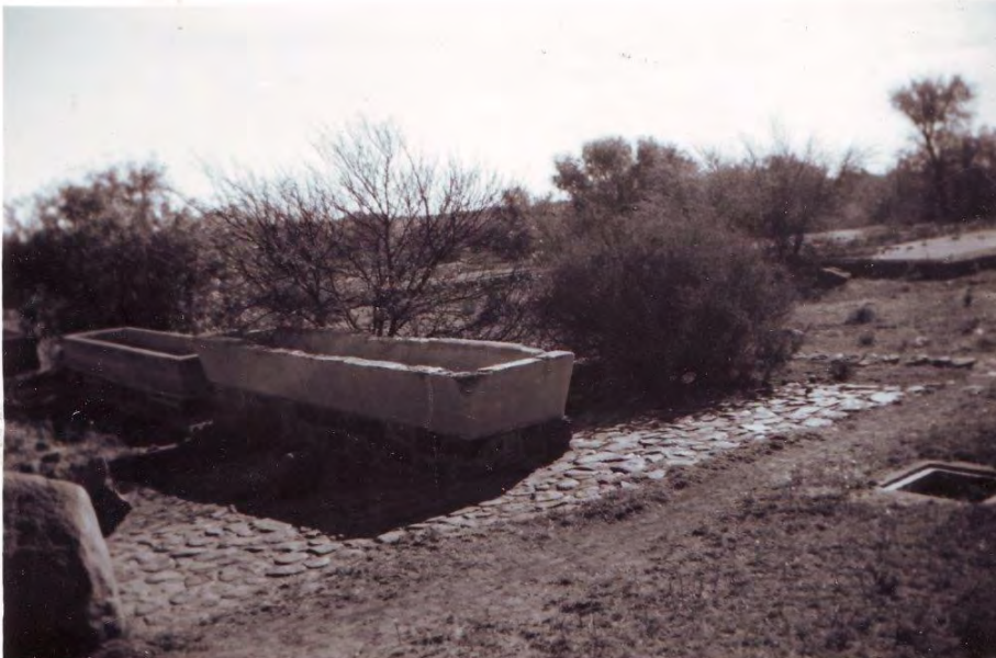
Figure 50: Photograph from the Free State Archives (VAB 8055) of the water troughs. Note the paving around the water troughs as well as the manhole on the right hand side of the photograph.
