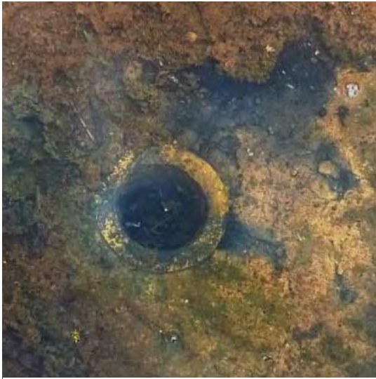
Figure 48: Picture of brass basin waste- trough was filled with water at the time
