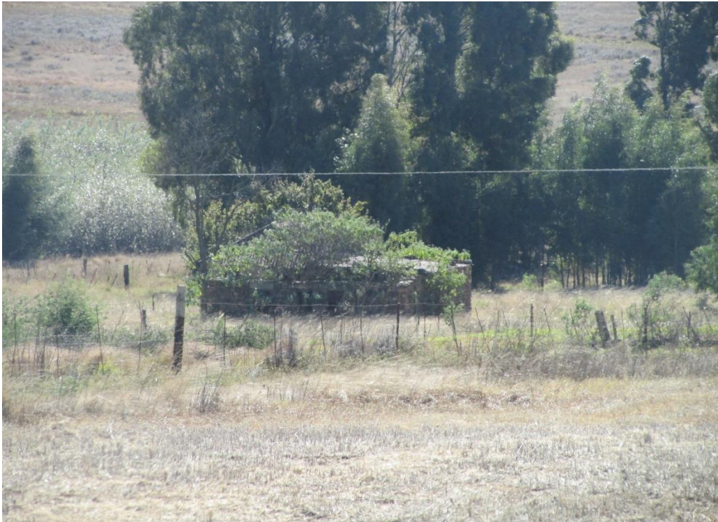
Figure 45: The sandstone structure at Site FS9.
