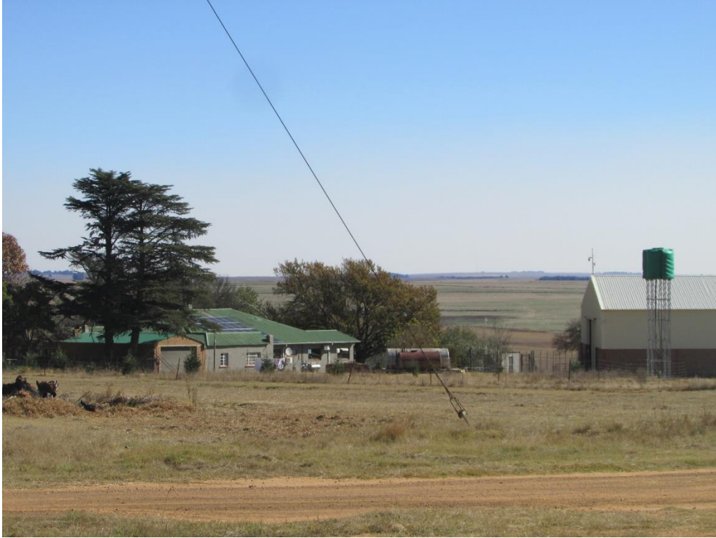
Figure 43: Partial view of Site FS7.
