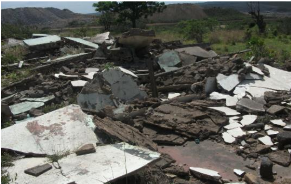
Figure 8: Remains of cement structure
