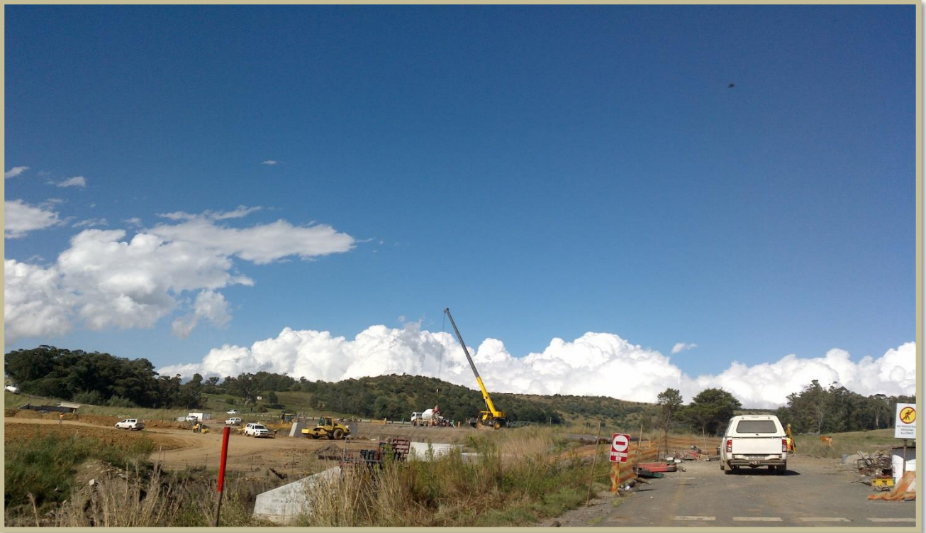
Figure 2 Current construction work
