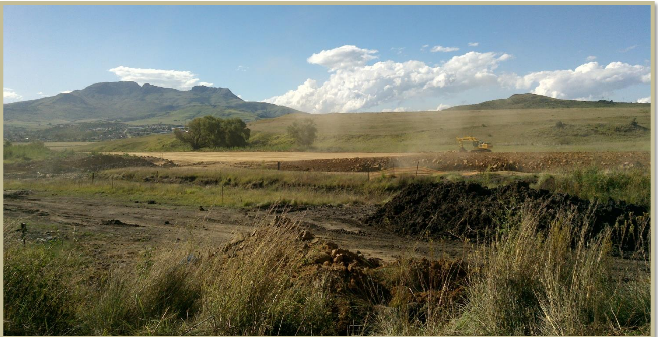
Figure 3 Current construction work
