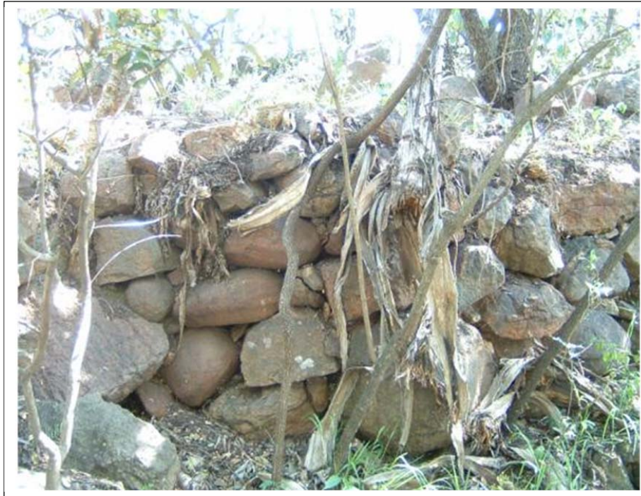
Figure 8- Close view of a stone wall in Site LIA01 reveals how small stones were used to wedge larger stones during the construction of walls (below).
