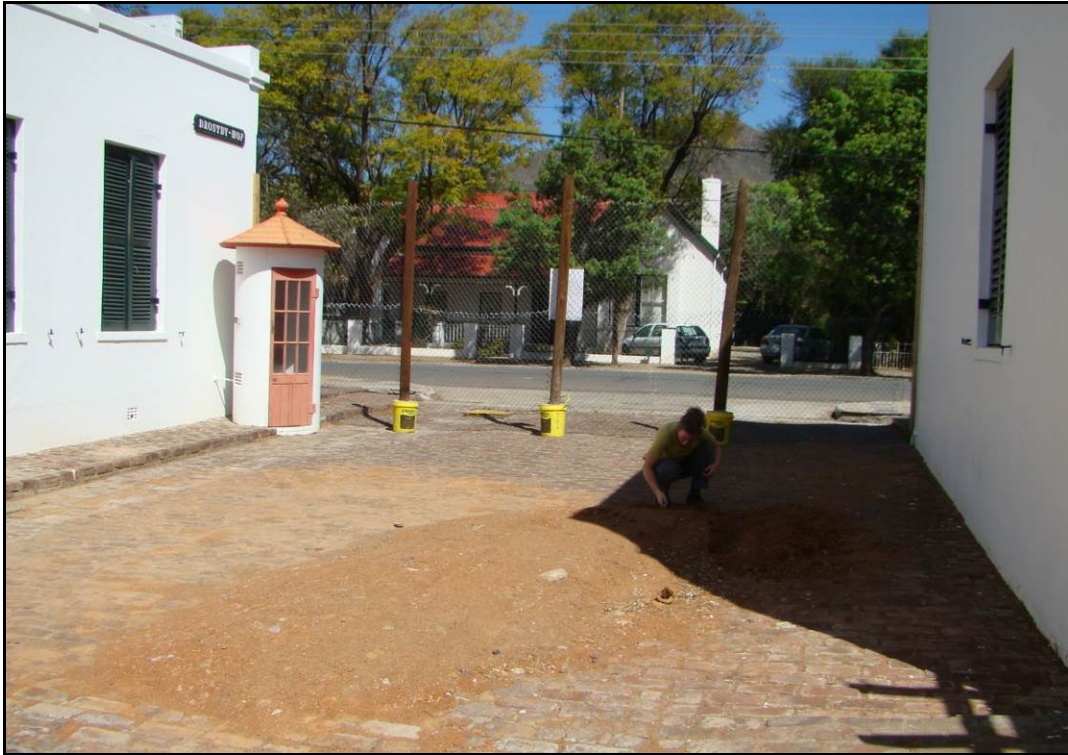
Figure 18: The location of the spoil heap at the Bourke Street entrance to Stretch's Court.
