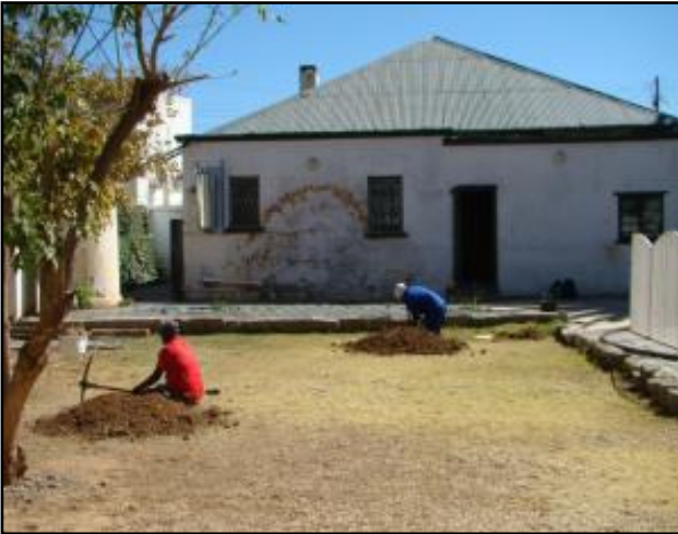
Figure 8: Excavating Test Pits 1 and 2.
