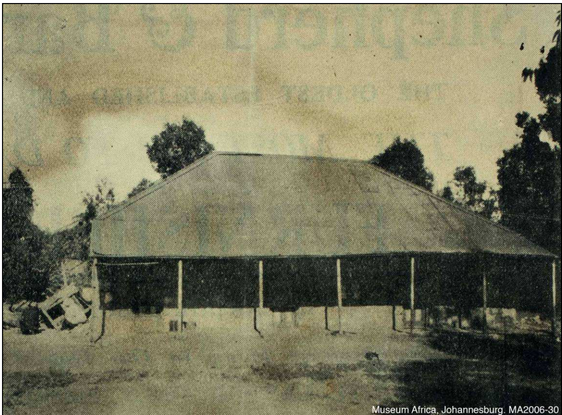
Figure 14 Photograph of the old stone building dating from the early 1890s that was located in an area referred to as Comet Plantation. The building was used for accommodation and as a mess-room (Museum Africa, Images Collection, MA2006-30).
