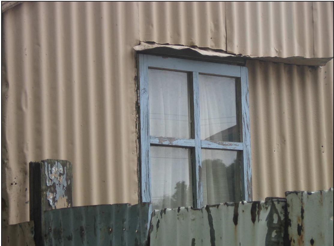
Plate 23 The original wooden window from an old corrugated iron outbuilding.
