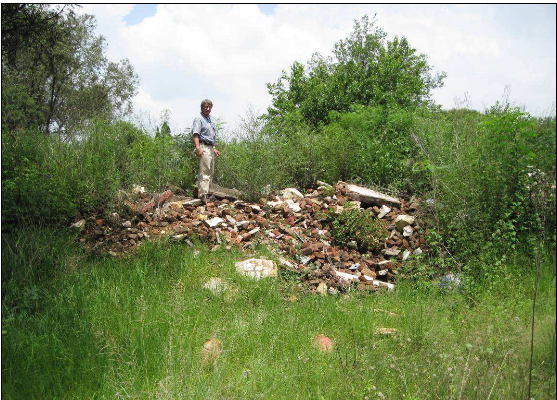
Plate 41 All that remains of what used to be the new married quarters known in this report as Building 6. The Kirkness brick alluded to in the report was observed here.
