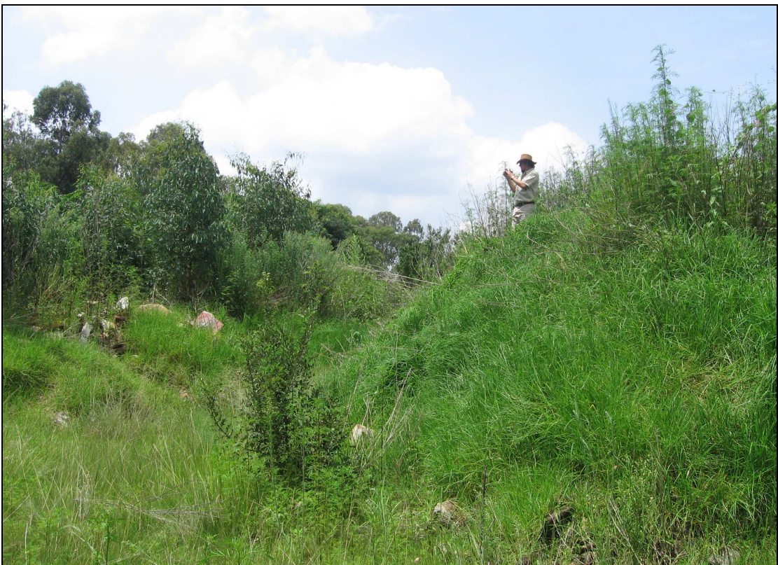
Plate 37 All that remains of what used to be the new married quarters known in this report as Building 5 is a large mound of rubble.
