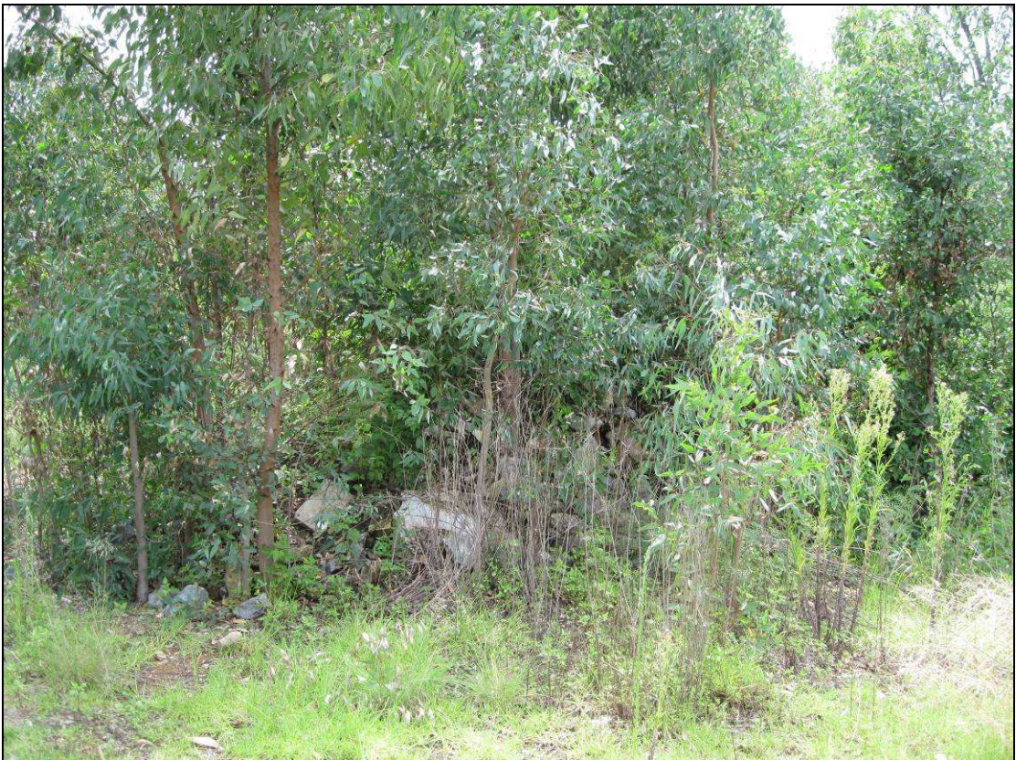
Plate 33 All that remain of Building 4 is this mound of rubble.
