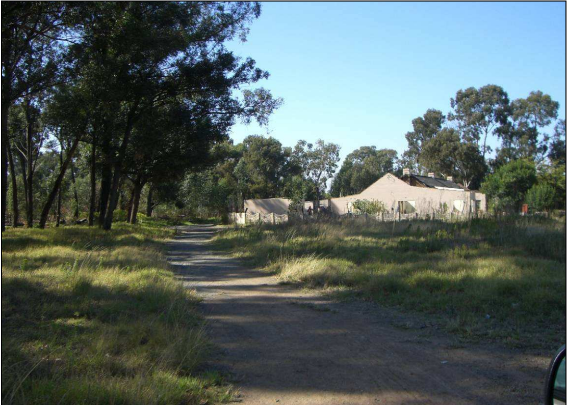
Plate 28 This image taken before or during 2007 appears to show the old married quarters known in this report as Building 4. The view is from the northwest.
