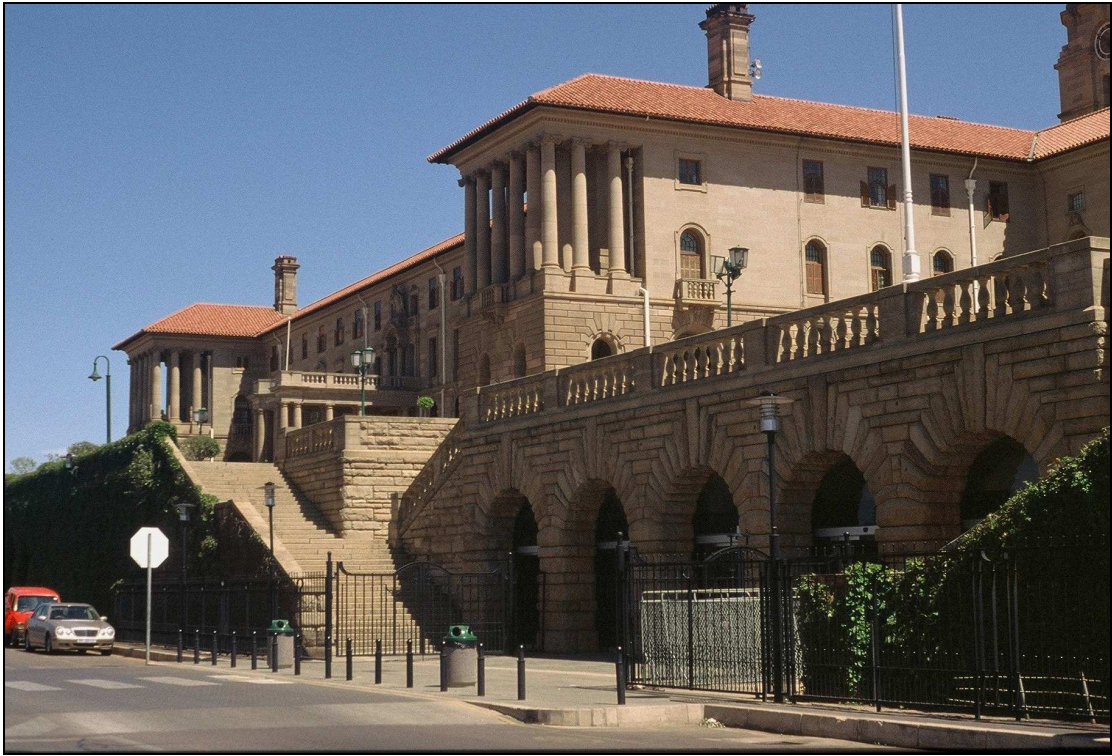
Plate 16 A similar pattern emerges in Baker's work with the simple rectangular floor plan pushed backwards by adding a pavilion at each side of the front elevation - here applied at the Union Buildings but also applied at the ERPM housing units in minute scale.
