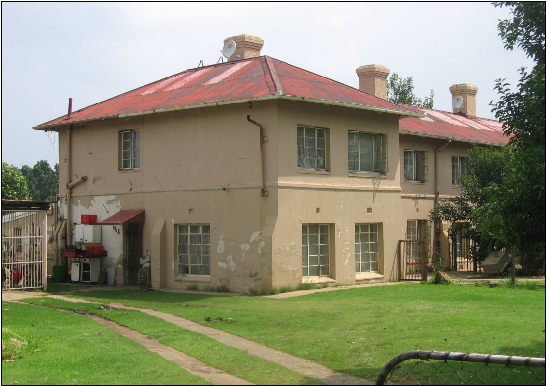
Plate 19 Corner elevation of one of the terrace buildings at ERPM with a slightly protruding pavilion and small buttressing element at its corner.
