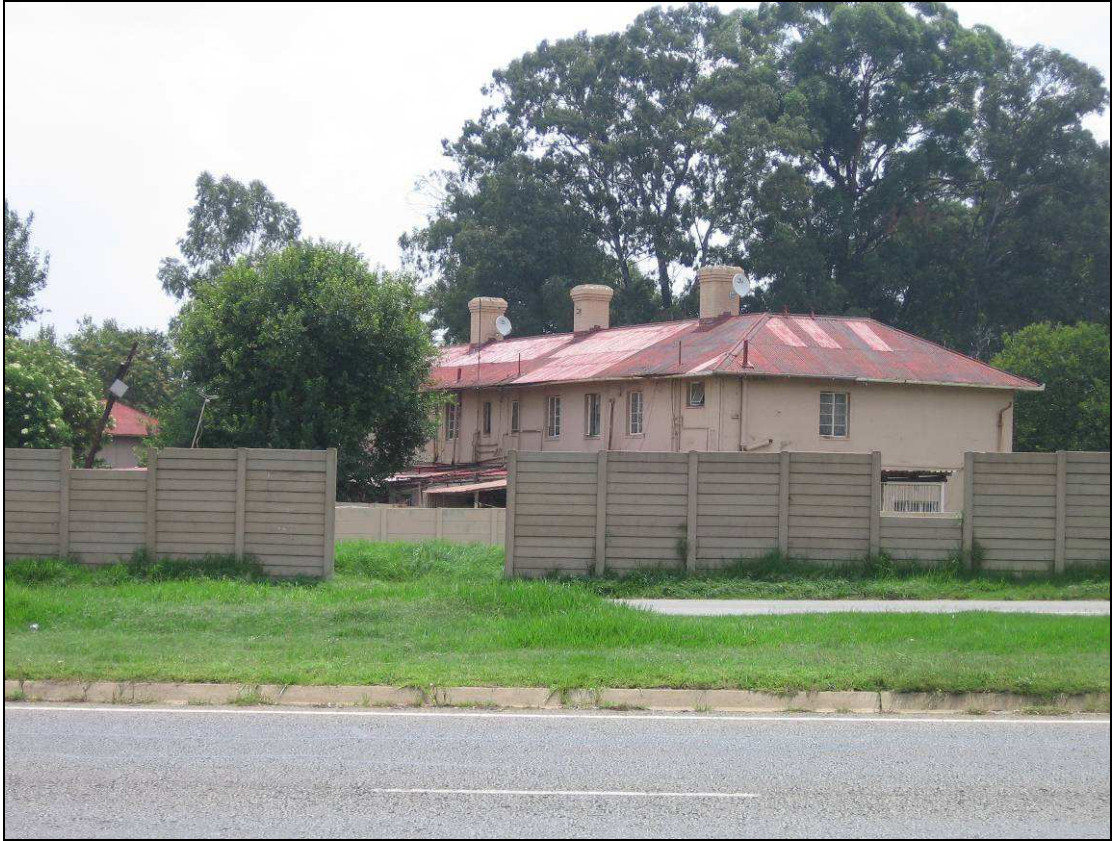
Plate 14 View from Rondebult Road towards the southern elevation (back elevation) of one of terrace buildings located to the west of the aforementioned road.
