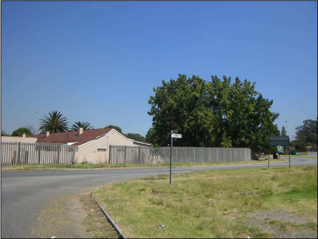
Plate 24 This image taken before or during 2007 appears to show the old married quarters known in this report as Building 1. The view is from the east.
