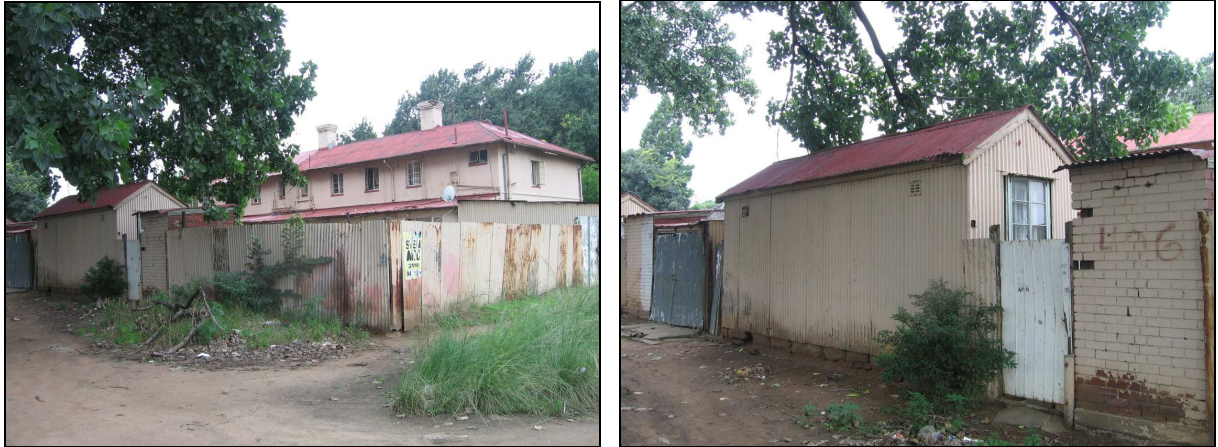
Plates 21 & 22 Exterior of backyard walling and small timber and iron outbuilding.
