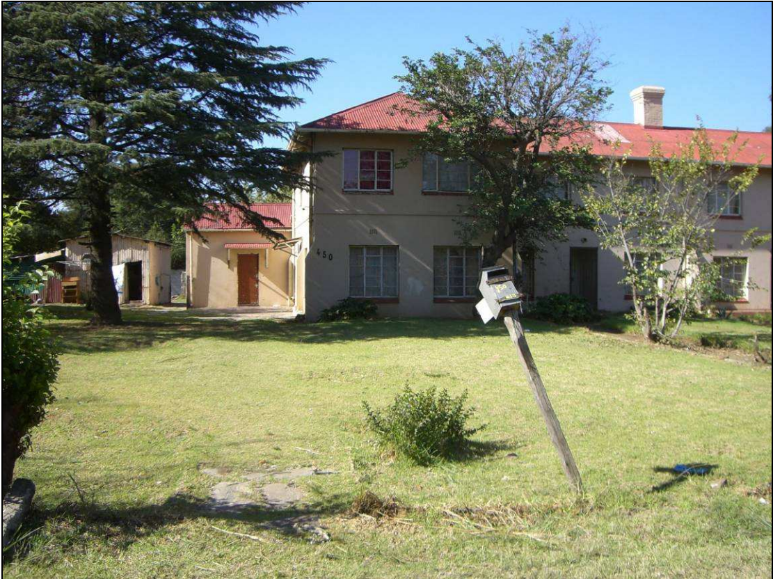
Plate 36 This image taken before or during 2007 appears to show the new married quarters building known in this report as Building 5.
