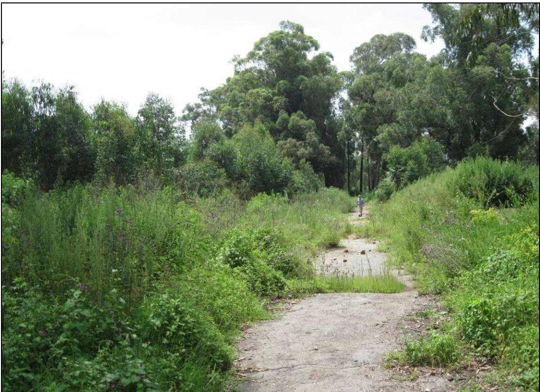
Plate 31 This image taken during 2010 shows more or less the same view as depicted in Plate 30. Note the marked difference between the two views with Building 4 completely destroyed and the overgrown state of the surrounding landscape.
