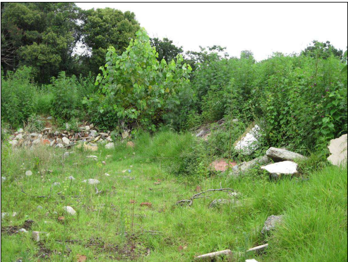
Plate 27 All that remains of what used to be the old married quarters known in this report as Building 2.
